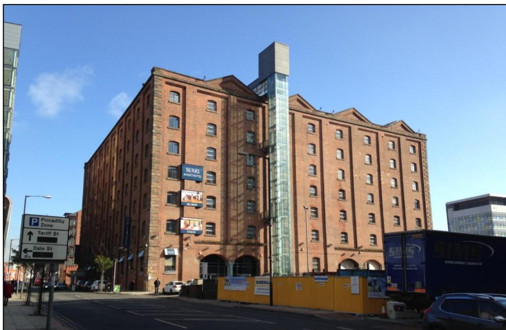
Figure 2.1: Ducie Street Warehouse from Ducie Street, south-west elevation
