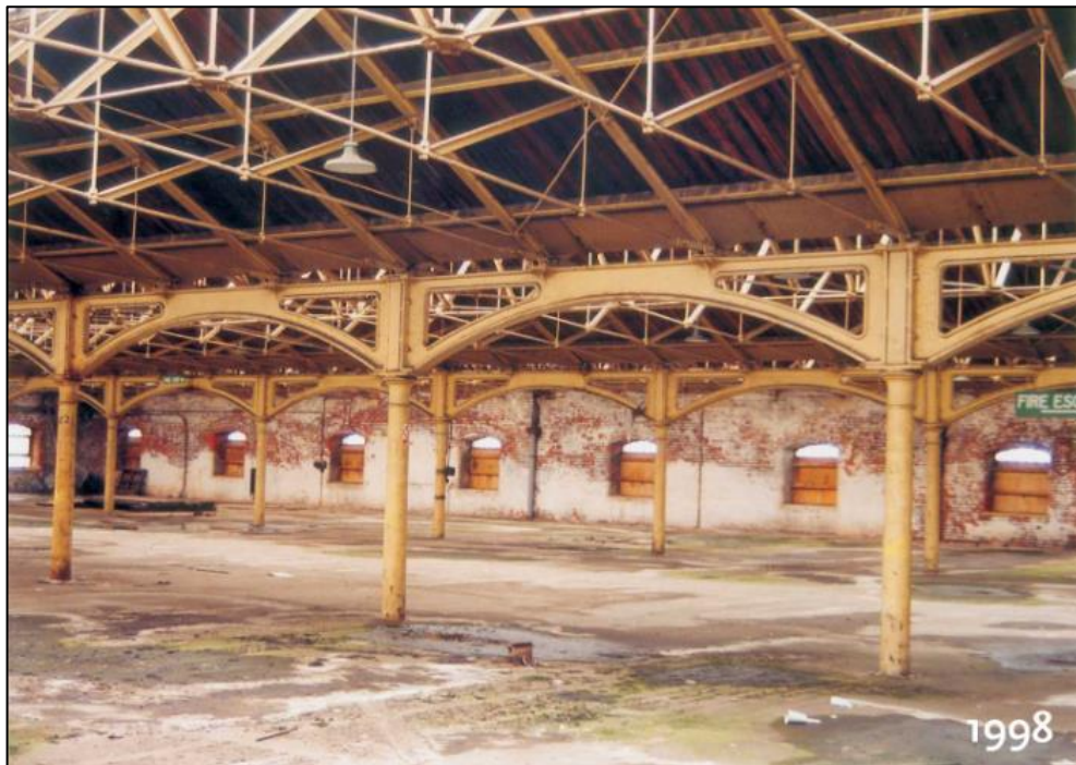
Figure 2.9: 1998 image of warehouse interior before conversion
