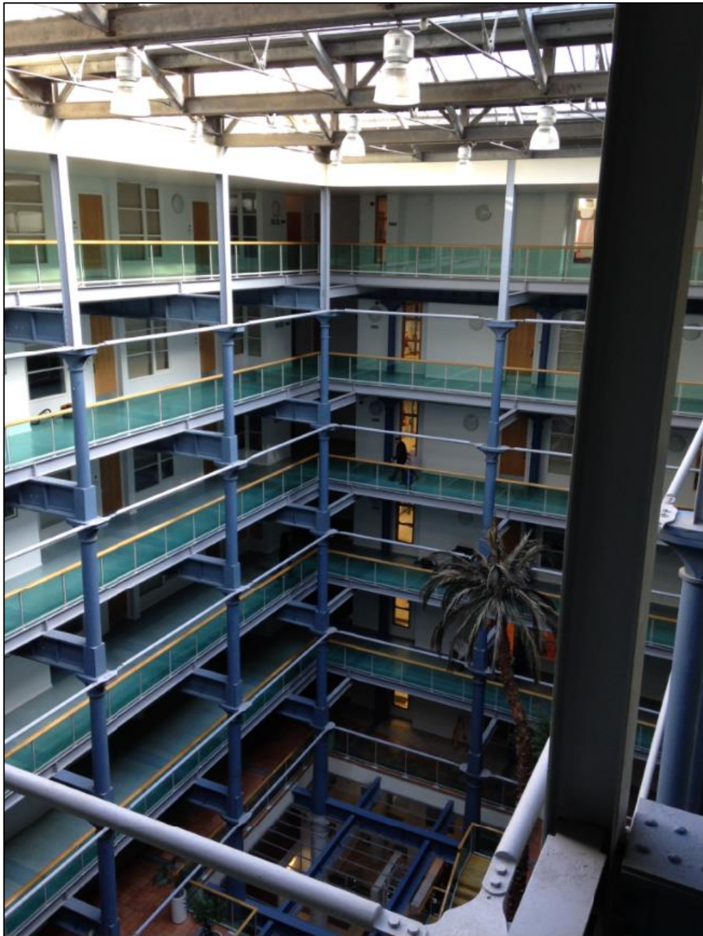
Figure 2.19: General view of atrium space
