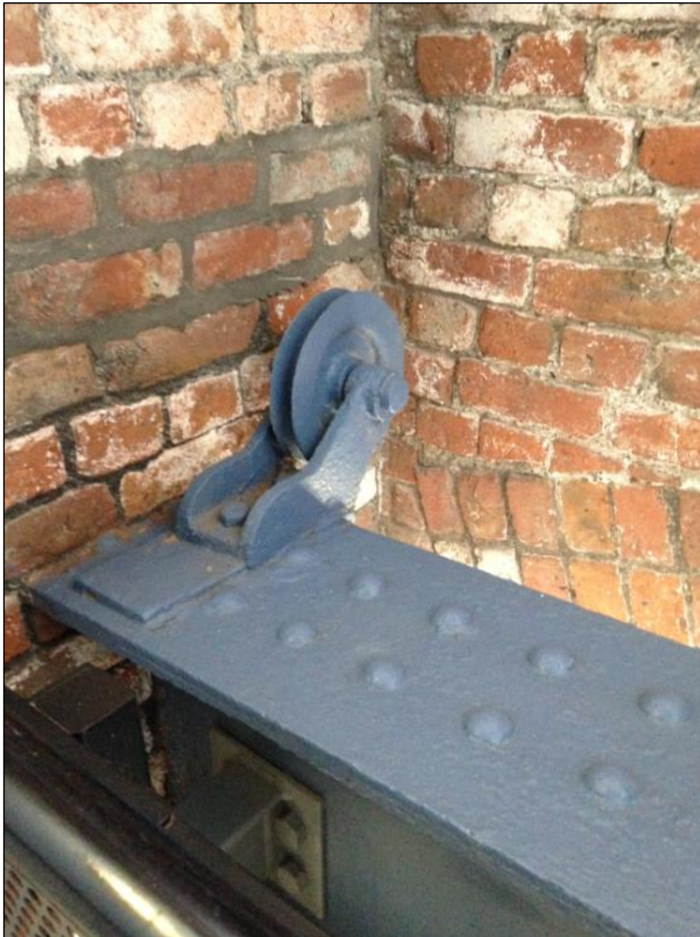
Figure 2.20: Historic hoist wheel, in modern staircase
