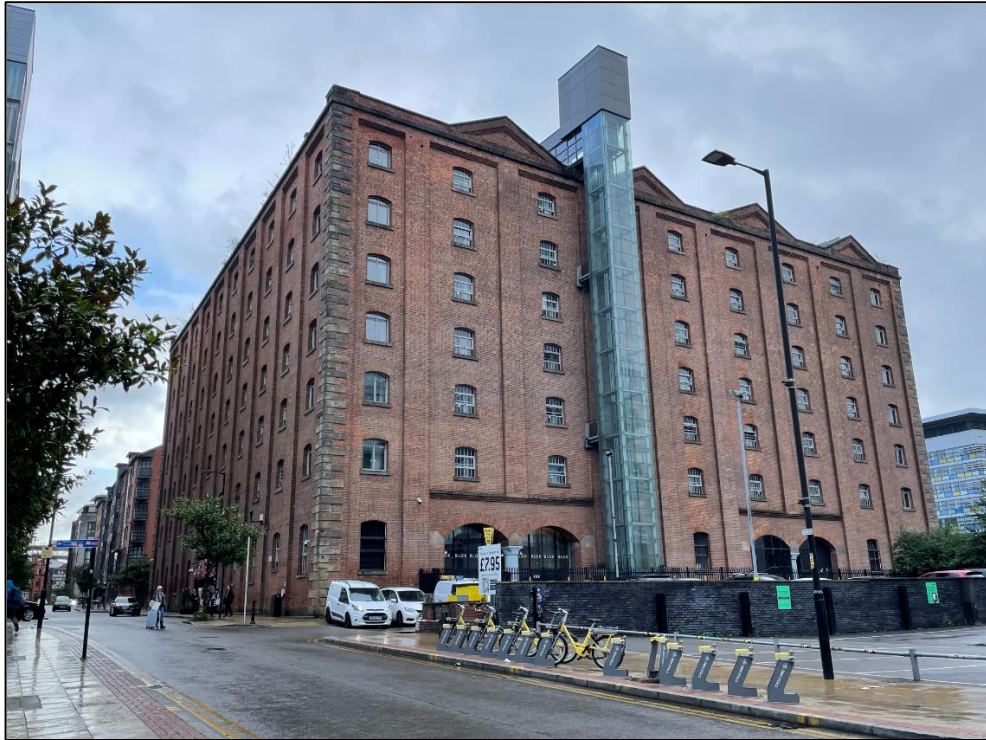
Figure 2.13: Ducie Street Warehouse from Ducie Street, south-west elevation
