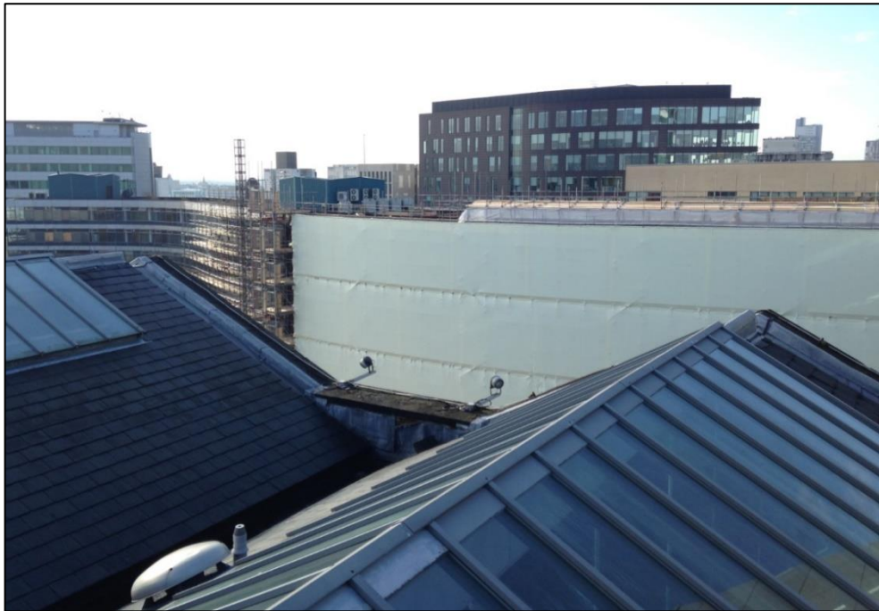
Figure 2.28: Gabled roof profile, with glazing ridge lights
