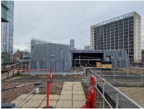
Ph.01 View looking North
