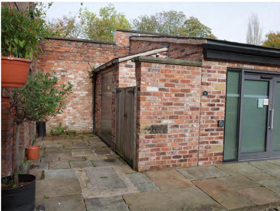
View 2 Looking towards storage area in north west corner of block. The small service area sits within the ownership of an adjacent tenant and would require legal agreements to enable use for equipment in an enclosure. Even if this was possible, the ducting and cabling required to 'join' the remote location to the Units 3 area would result in additional unacceptable intrusion on the listed fabric and the setting.
