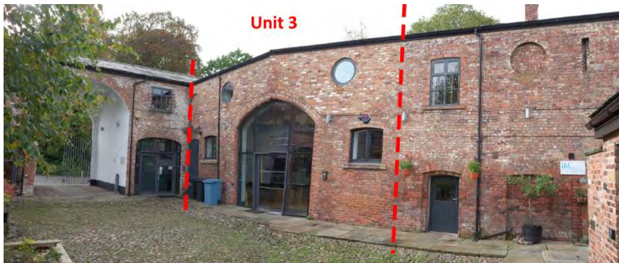
Courtyard looking towards south west corner with limited extent of Unit 3 ownership indicated by broken red lines.
