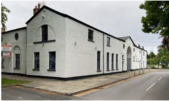
South Elevation of the Stable Block.
