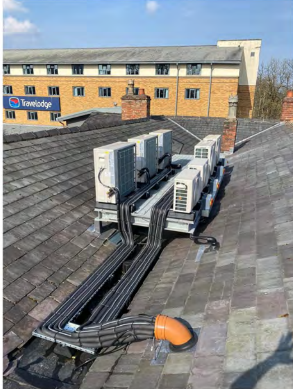
Views at roof level of the hidden installed air handling equipment and discrete cabling.
