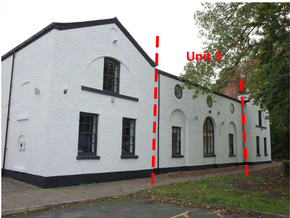
View 2 Looking towards west elevation.
