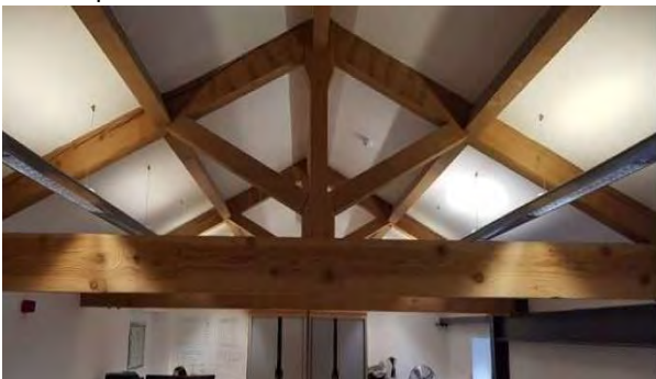
Replacement roof trusses from 2002 repairs/conversion.
