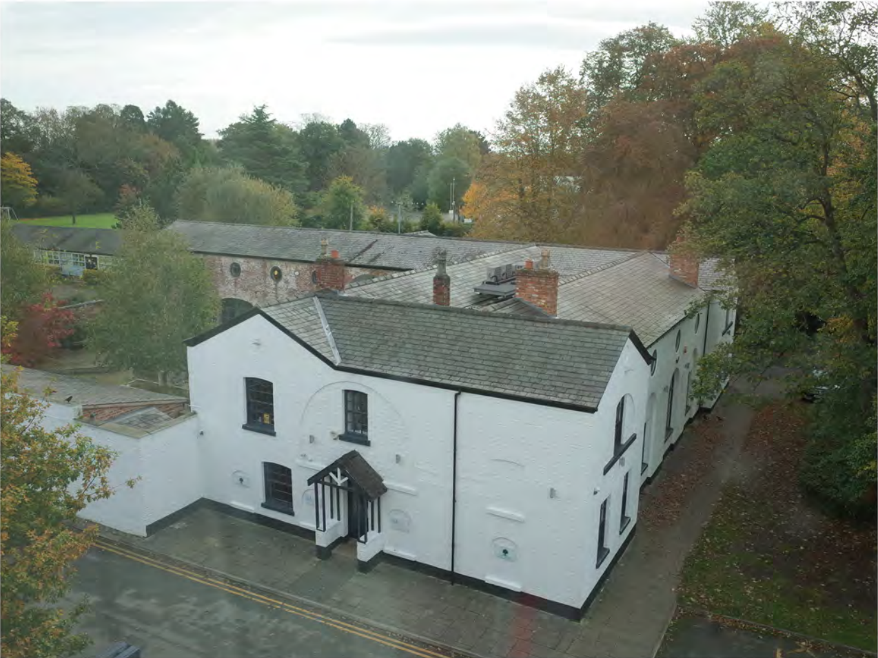
View of the equipment painted in slate grey (RAL 7015) to match the slate roofing finish.
