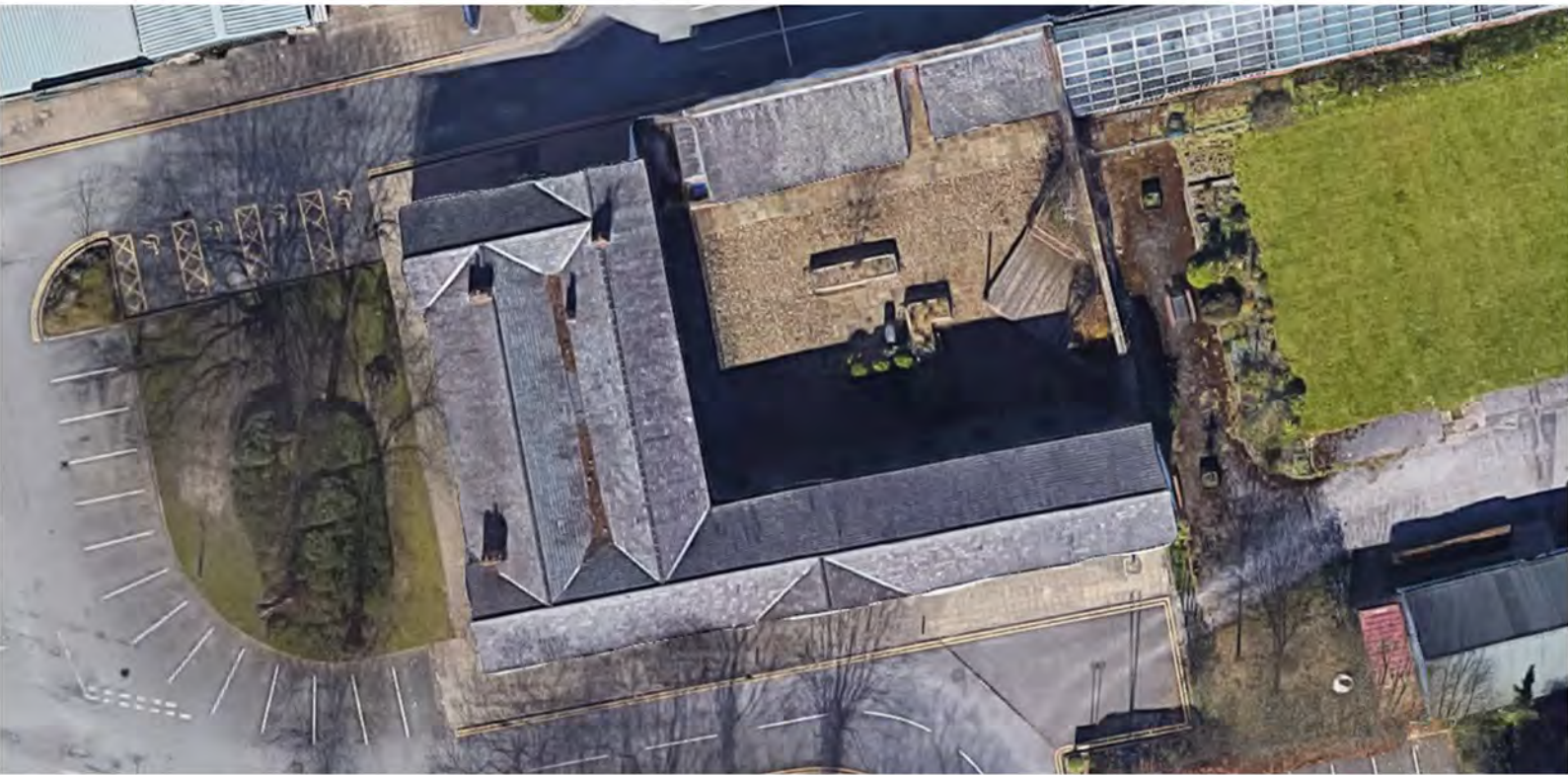
Aerial view of roof valley prior to installation of air handling equipment.
