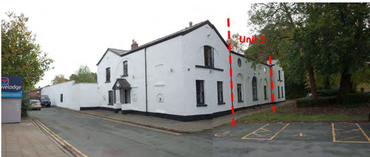
North and west external elevations with limited extent of Unit 3 ownership indicated by broken red lines.
