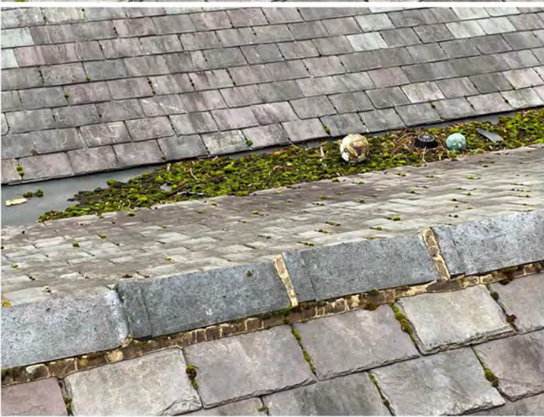
Roof valley condition.
