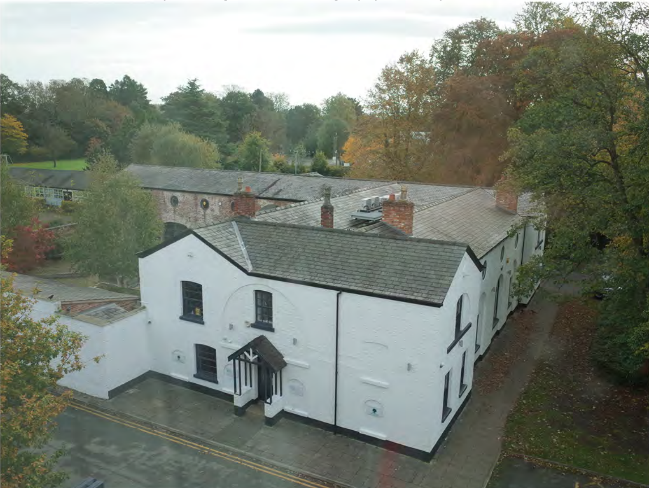
View of installation from the 4th floor bedrooms of the adjacent Hotel.
