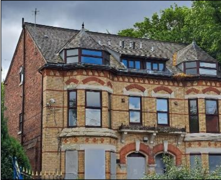
Photograph 4 showing the front elevation
