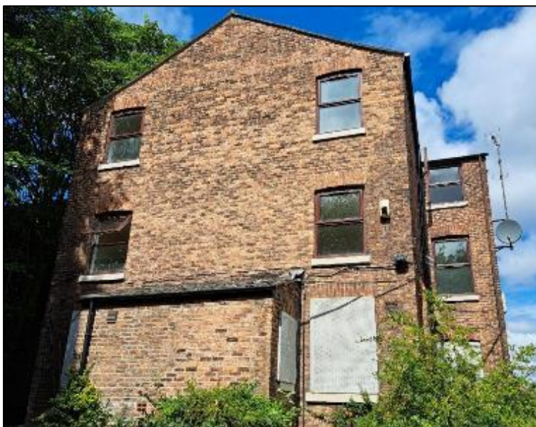
Photograph 7 showing the rear elevation and an open window
