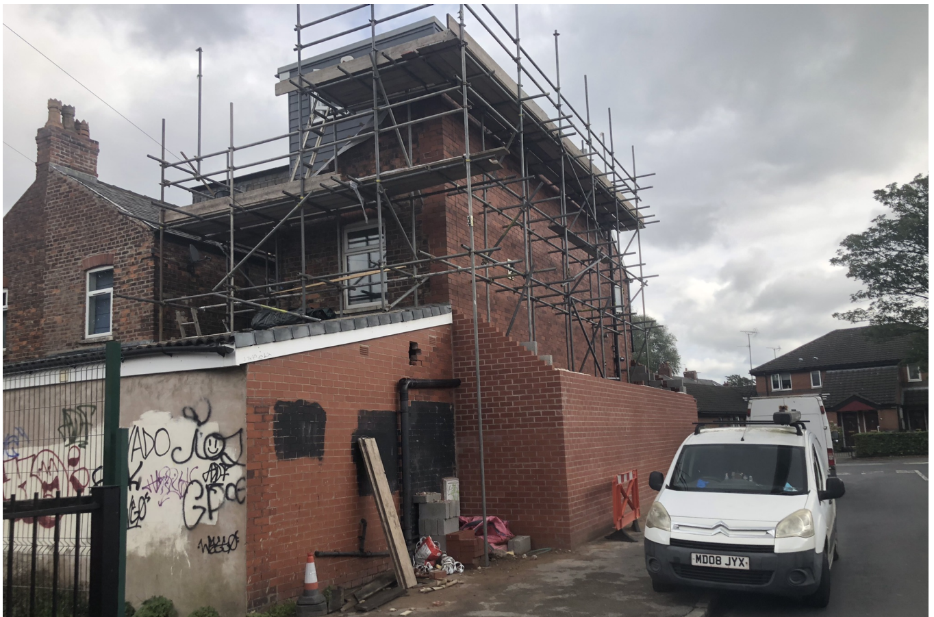
Figure 3. View of rear and side of property.
