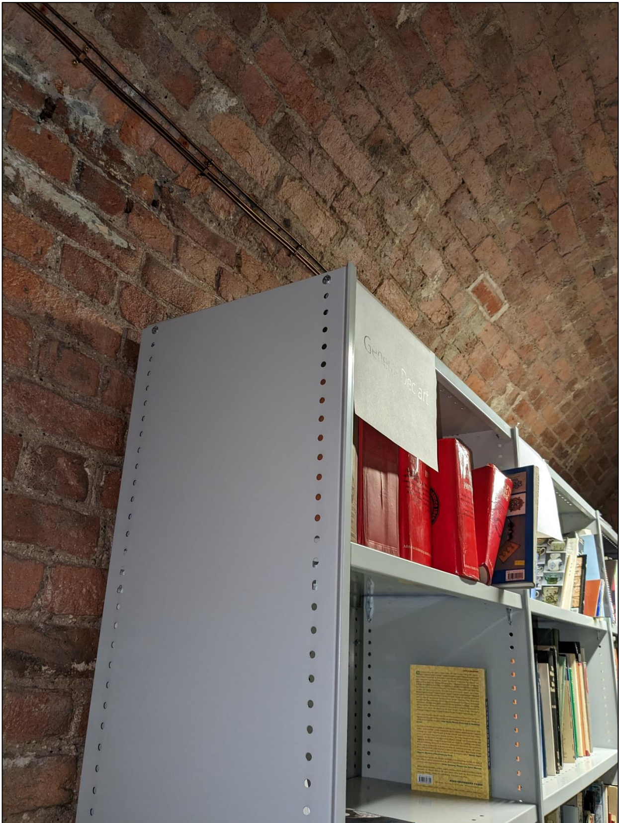
Appendix 6: A view of the shelf, above which the hole enters LG20, this eye-level shot demonstrates the minimal impact the planned installation of LGAP2 will have on the buildings historic character.
