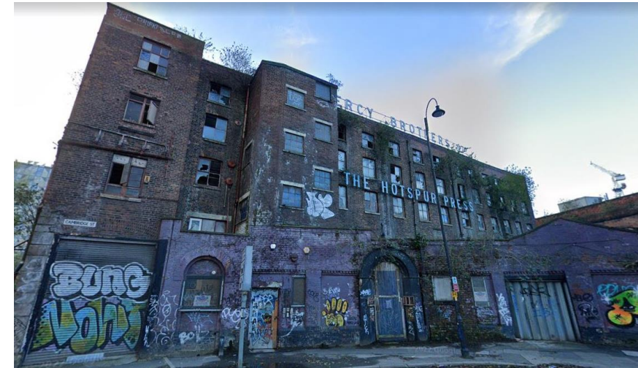
Figure 7 Existing front façade.
