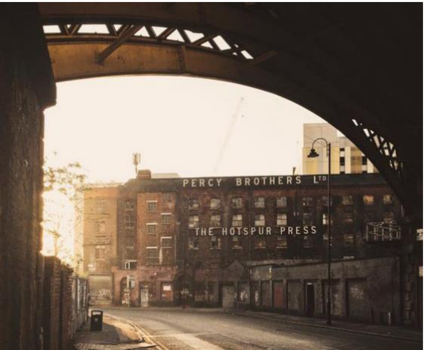
Figure 3 Image of the existing building.
