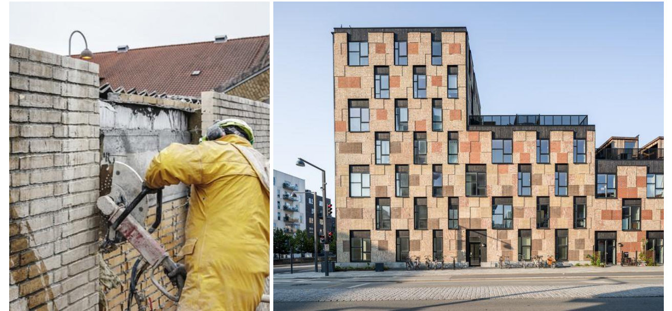
Figure 10 Reuse of existing brickwork in a modular panellised format at the Resource Rows project by Lendager.
