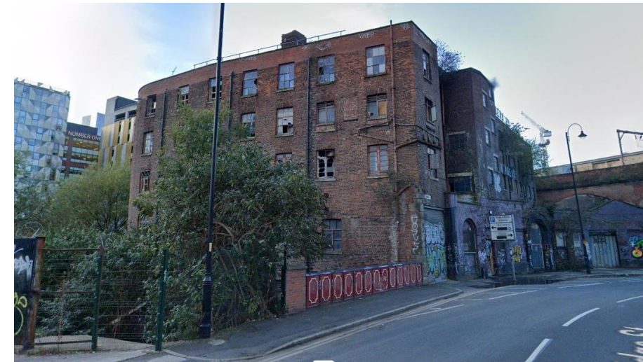
Figure 8 Existing side façade.
