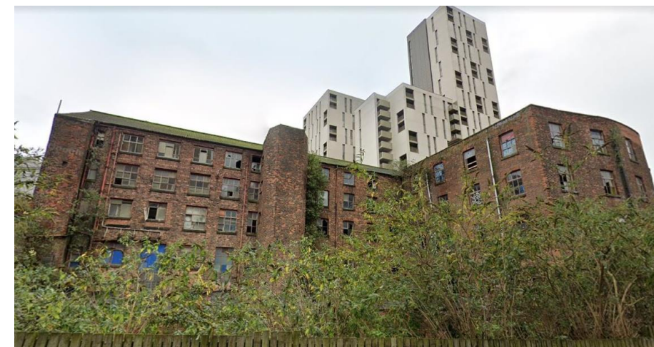
Figure 9 Existing rear façade.
