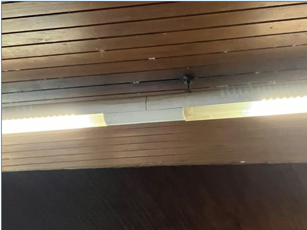
Figure 9 - Existing strip lighting located central to station canopy.
