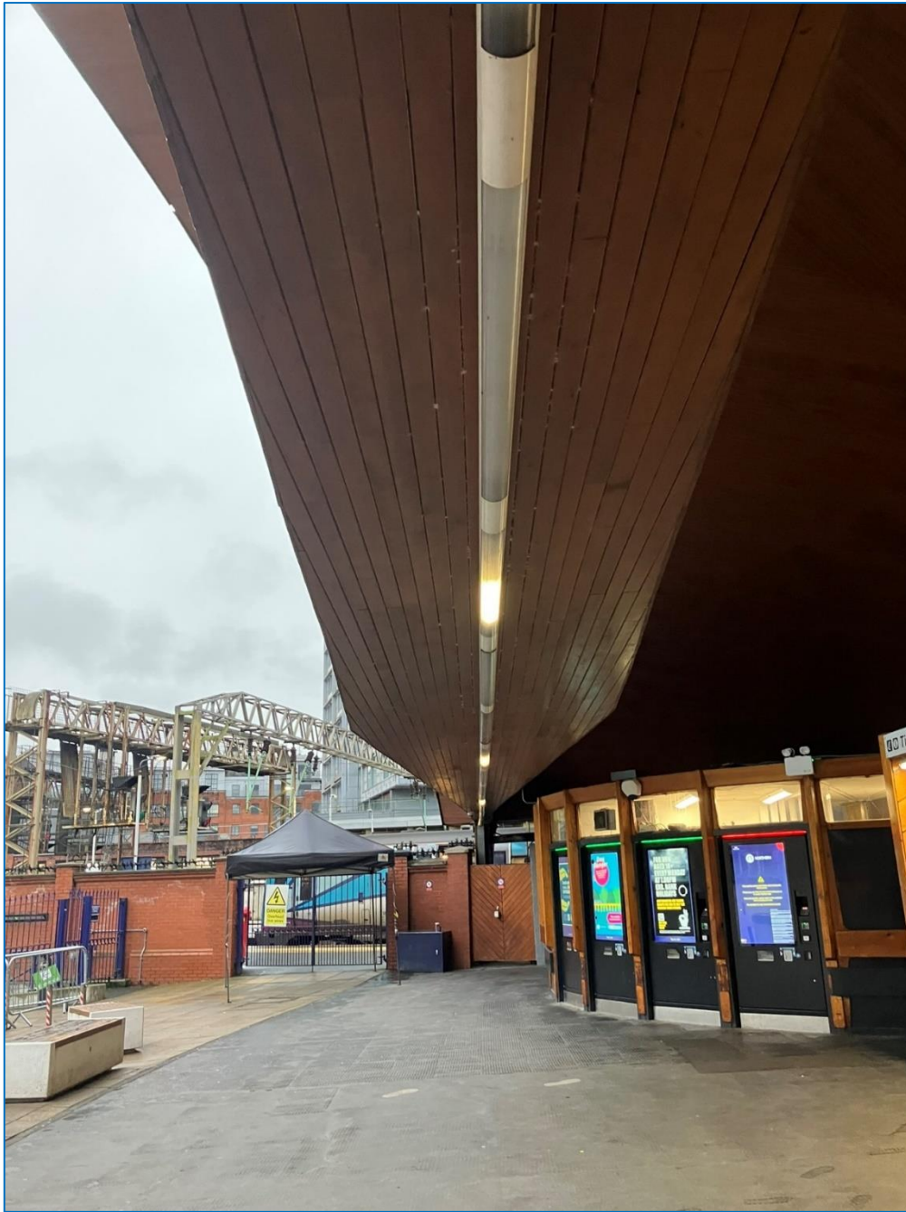
Figure 10 - Strip lighting located central to station canopy width (19/12/2023)
