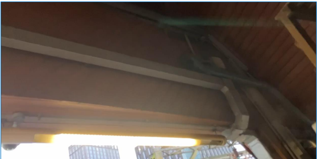
Figure 12 - Existing CCTV camera, associated trunking on underside of canopy and additional trunking on rear face of canopy (taken from building side)
