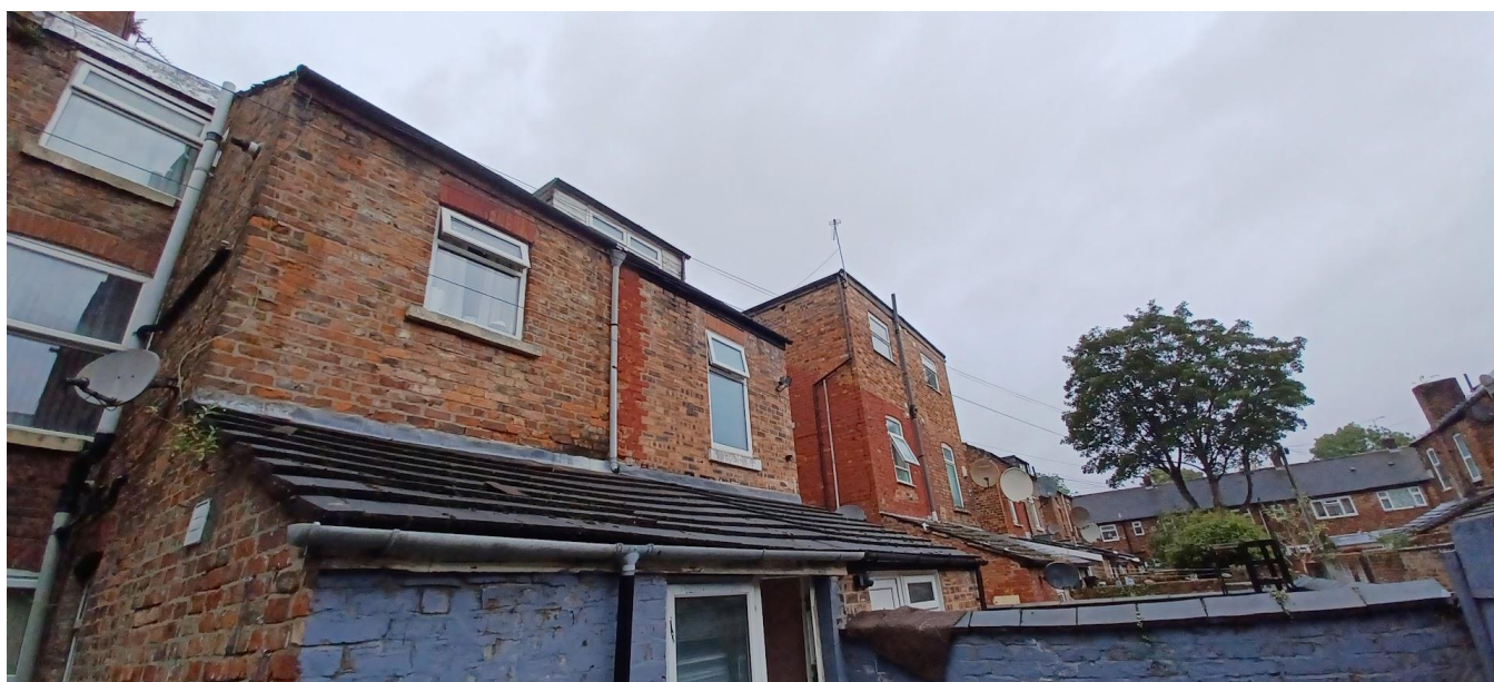
Figure 5. Application property with No.7 and No.9 Bedford Avenue visible in background.
