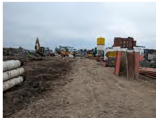
Photo 7 – Construction across much of site
