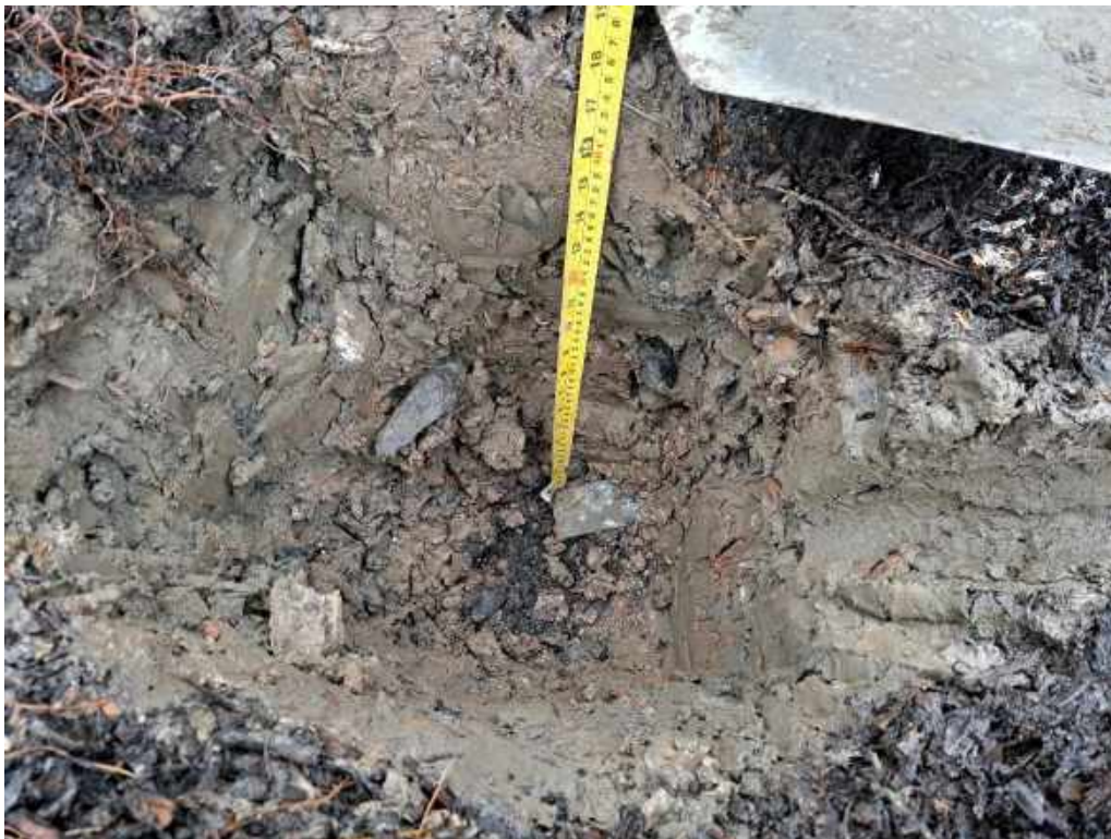
Photograph 8 VP01 showing thickness of cover system.
