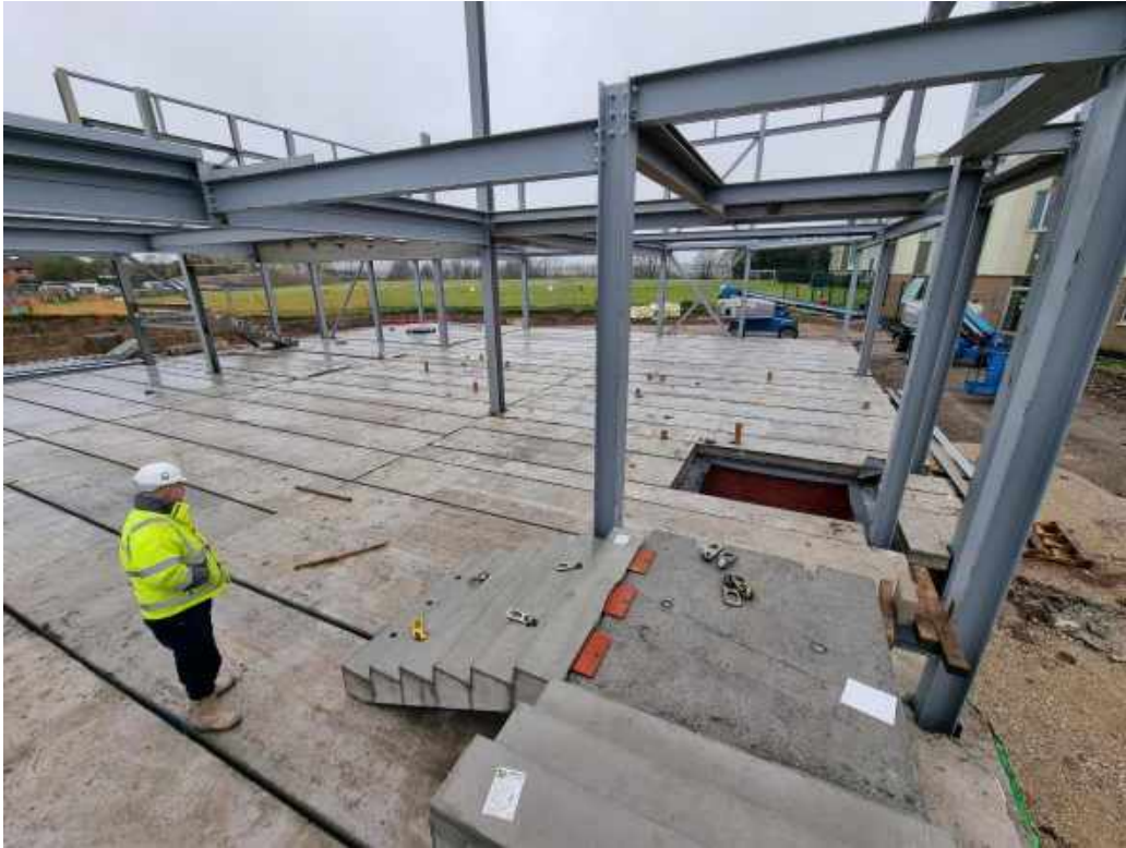
Photograph 1 Installation of steel frame and suspended floor 04/04/2022 (photograph supplied by client).
