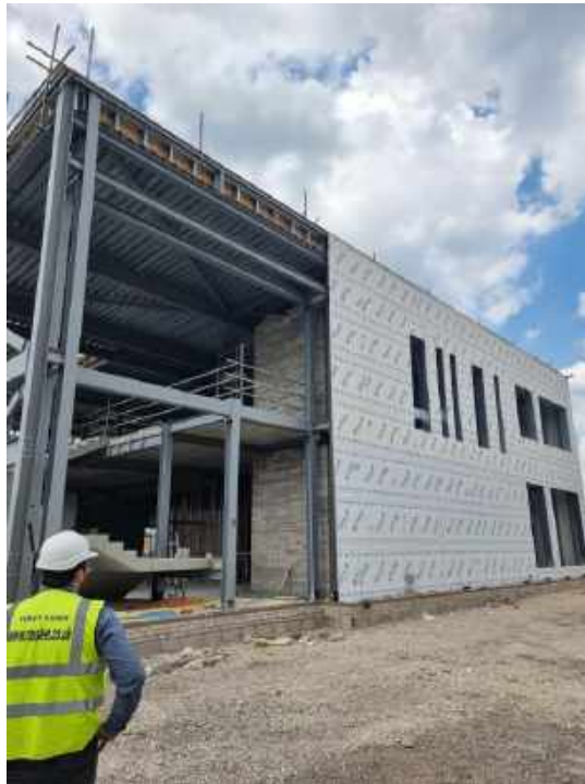
Photograph 4 External cladding of new building 23/06/2022 (photograph supplied by client).
