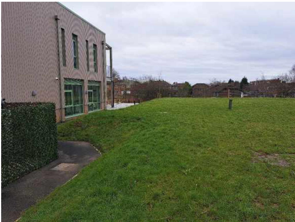
Photograph 6 Grassed attenuation tank to the west of the structure.
