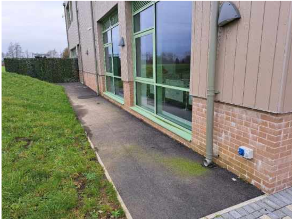
Photograph 25 Western face of new building.
