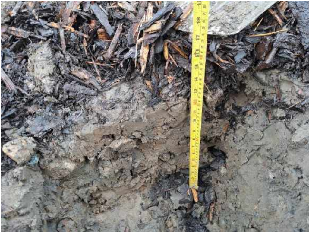
Photograph 11 VP02 showing thickness of cover system.
