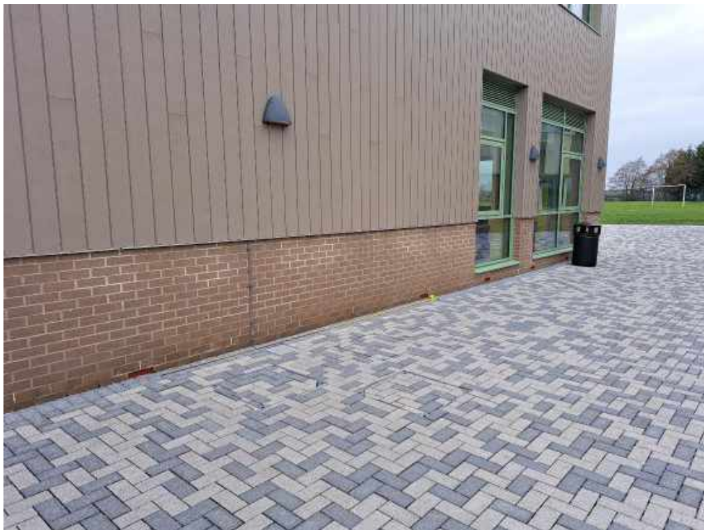
Photograph 26 Eastern elevation with periscope vents visible.
