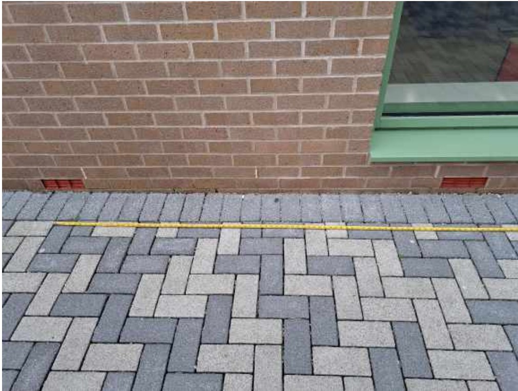
Photograph 27 Vents at 1.8m centres to eastern elevation.
