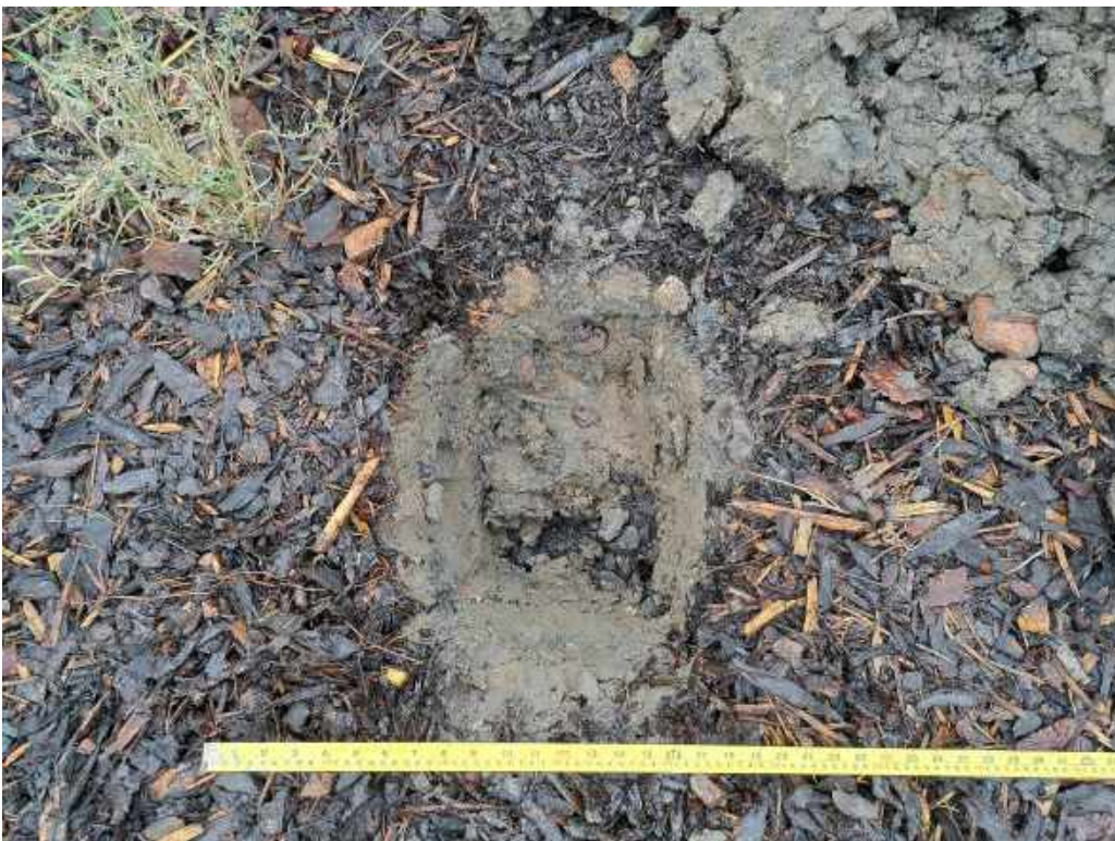
Photograph 10 VP02 – concrete obstruction in upper half of pit.
