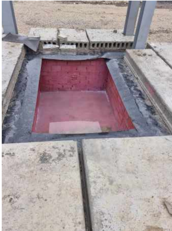
Photograph 3 Detail of membrane beneath suspended floor 04/04/2022 (photograph supplied by client).
