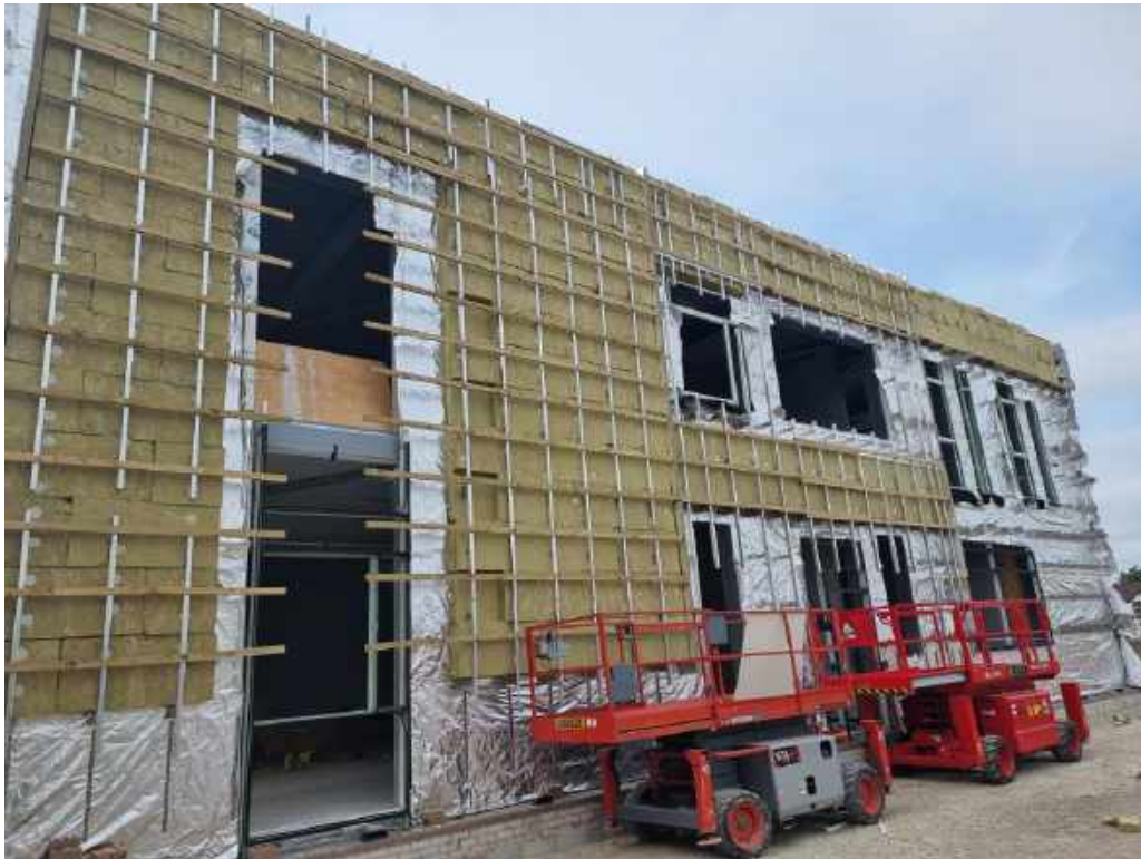
Photograph 5 External cladding of new building 20/07/2022 (photograph supplied by client).
