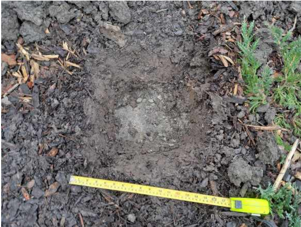
Photograph 13 VP03. Compacted gravel visible at base of pit.
