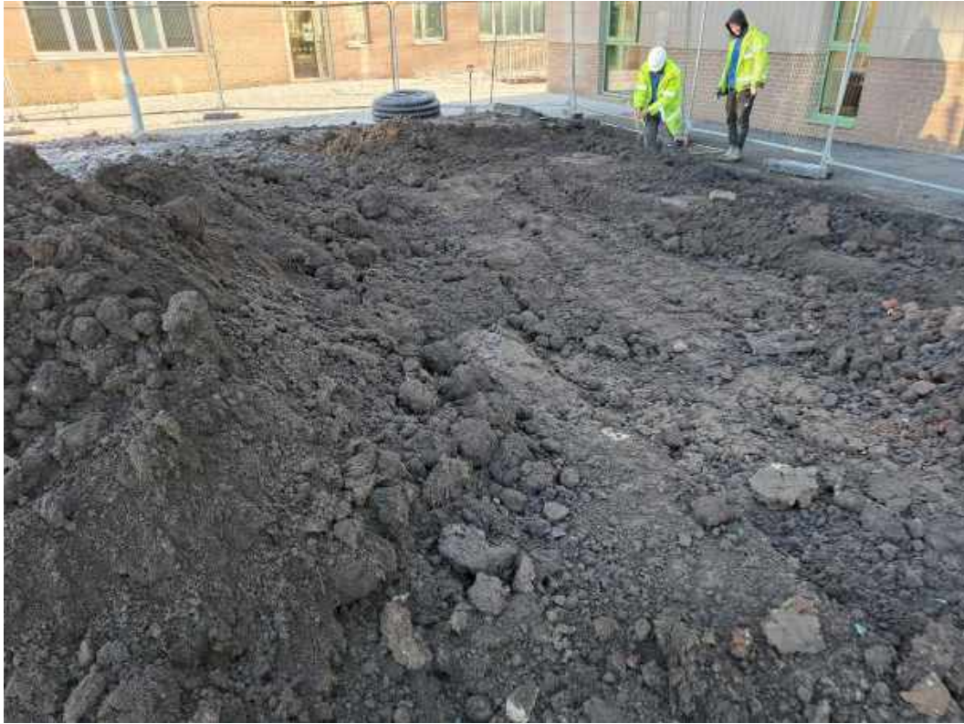
Photograph 3 Placement of cover system soils to north of new building (08/12/2022).
