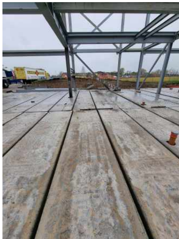
Photograph 2 Installation of steel frame and suspended floor 04/04/2022 (photograph supplied by client).
