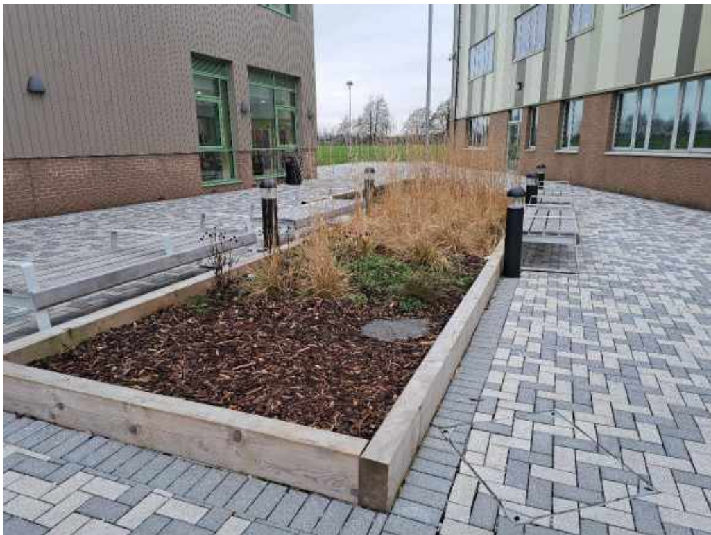
Photograph 4 Raised planter to east of structure before additional topsoil capping.
