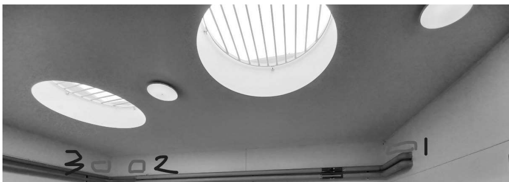
Appendix 18: Location of Hole 3 as seen from Room B01–GF-009.
