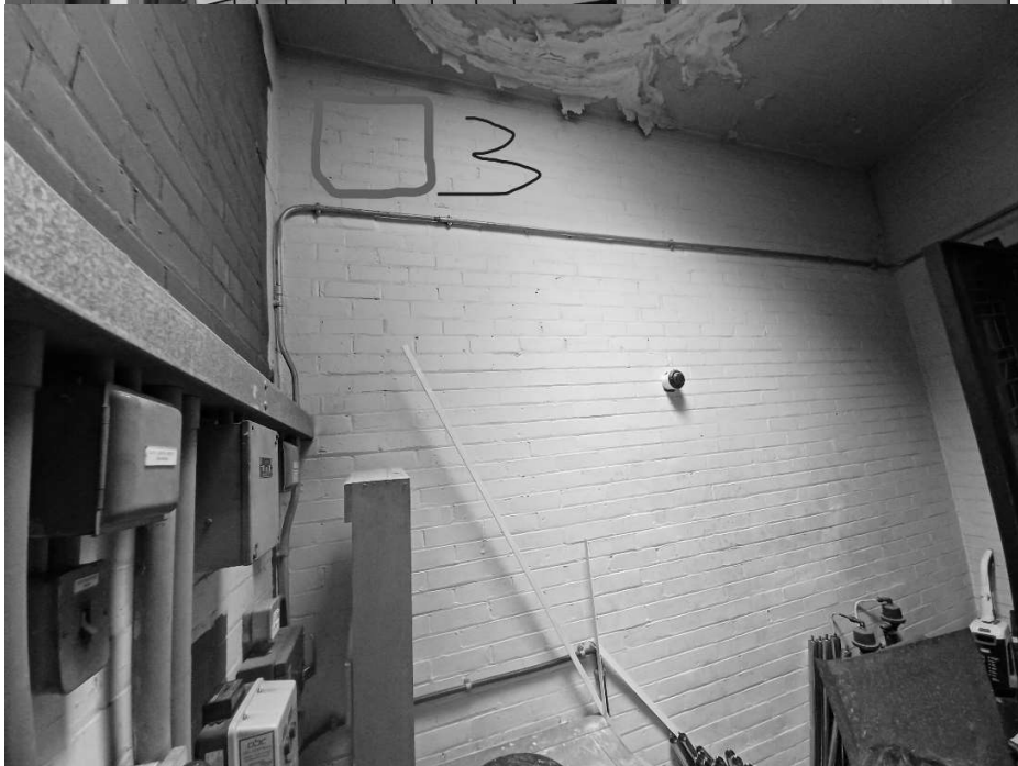
Appendix Location 2 and as seen Room 011.
