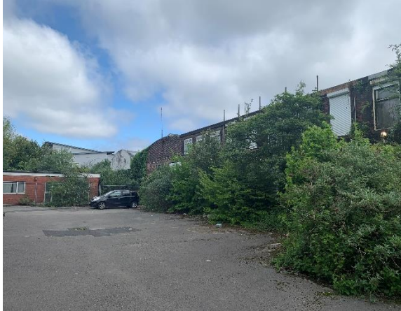
Photograph 5 – Hardstanding to the west of building B5
