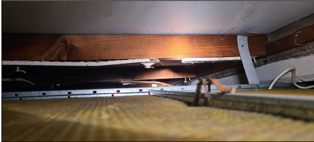
Plate 11. Space between the suspended ceiling and the insulated board under the sheet metal roof
