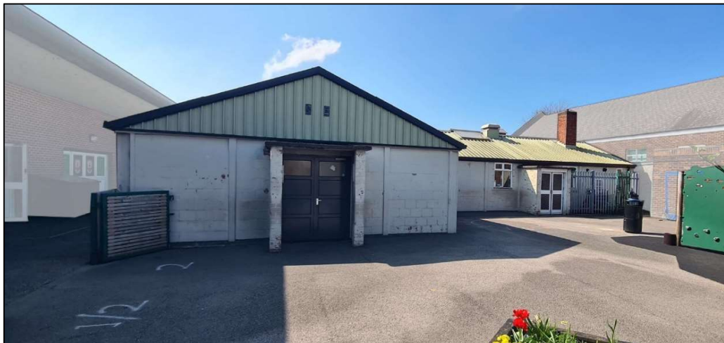
Plate 1. The north aspect of the building (adjacent buildings greyed out)
