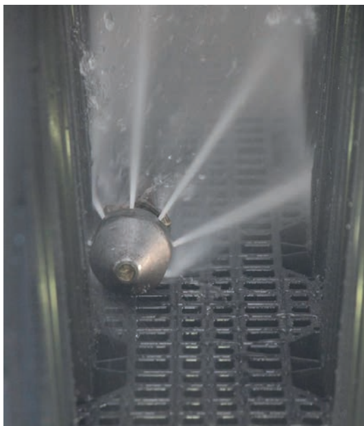
Figure 12 - Jetting nozzle flushing the system
