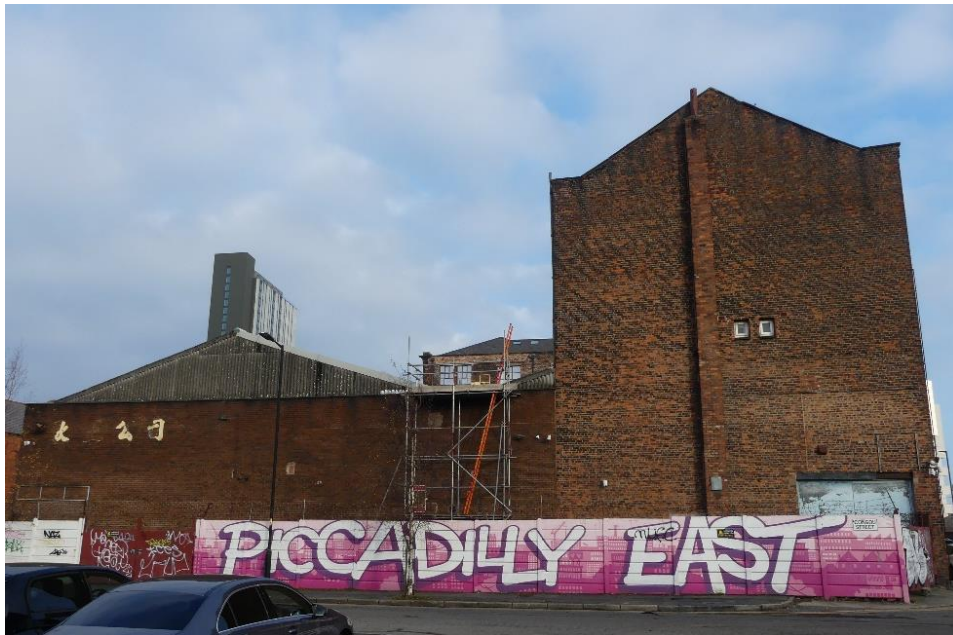
Figure 1.10: The southern elevation of the application site adjoining the single-storey warehouse
