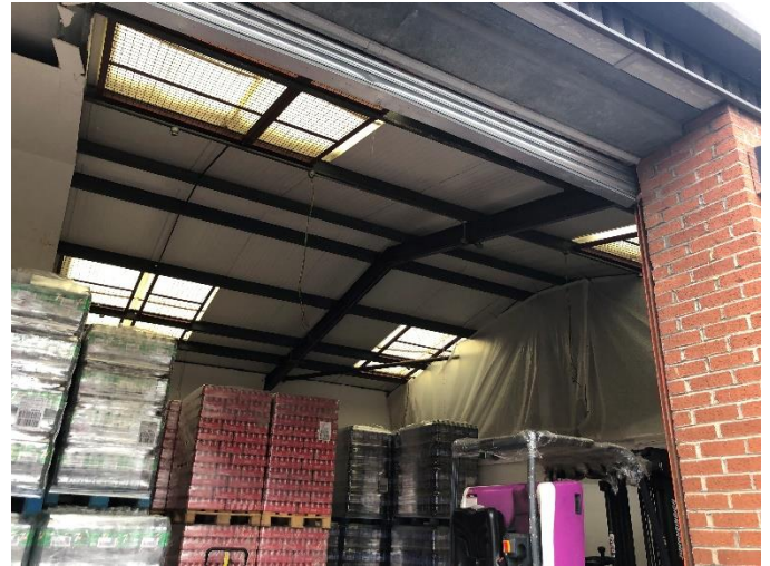
Figure 2-10 Illustrating how the buildings are open to the roof and include lighting panels
