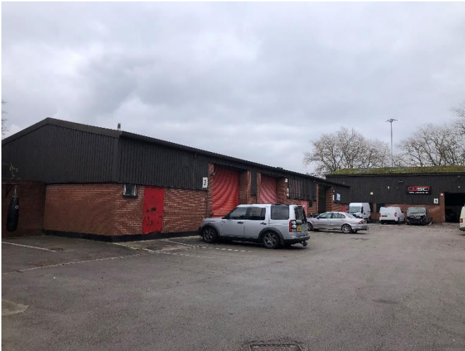
Figure 2-9 The typical construction type of buildings B13-17.
