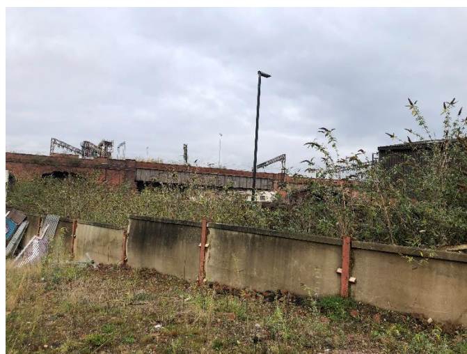
Figure 2-6 An area of dense buddleia growth between two fence lines in the western area of the site, adjacent to Hoyle Street
