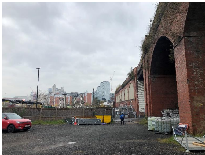
Figure 2-4 The northern area of the site, currently in use for occasional car parking and storage within the arches.
