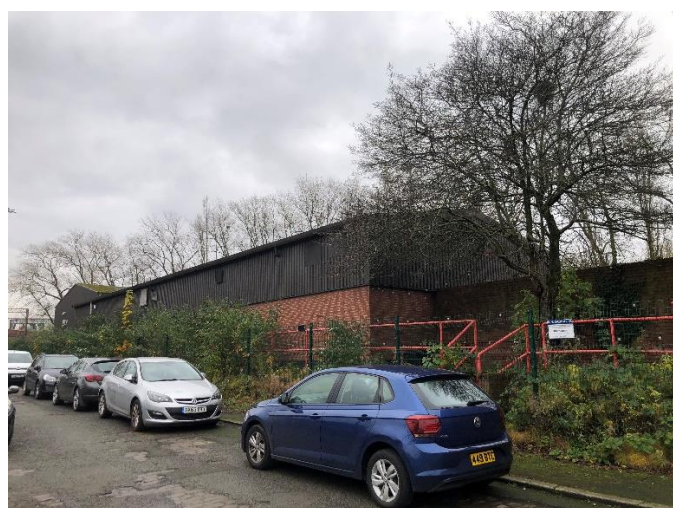
Figure 2-7 Vegetation growth, including a single semi-mature tree, along the building area boundary with Rachel Street
