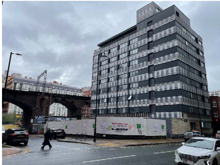
Figure 1.3: Views towards the Site from the junction of Charles Street and York Street; the Site and hoarding visible in the foreground.
