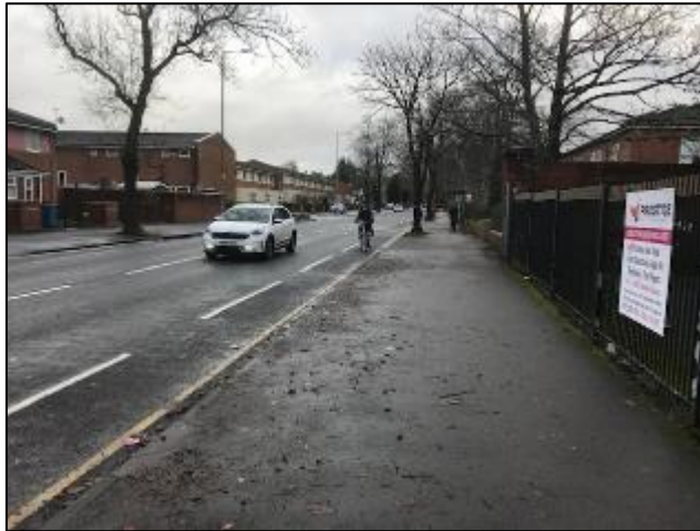
Plate HTN7 - Advisory Cycle Lane Infrastructure on A5184 Plymouth Gove (looking south east)
