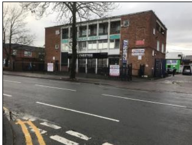
Plate HTN3 - Plymouth Grove Application Site Frontage & Access Driveway
