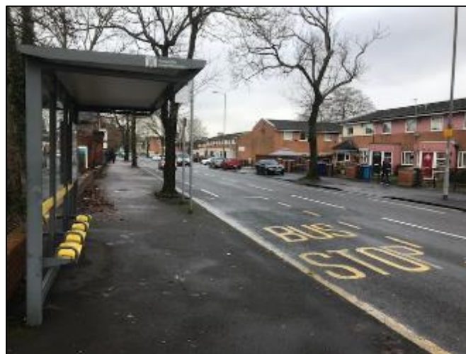
Plate HTN8 Westbound Bus Shelter Infrastructure to A5184 Plymouth Grove
