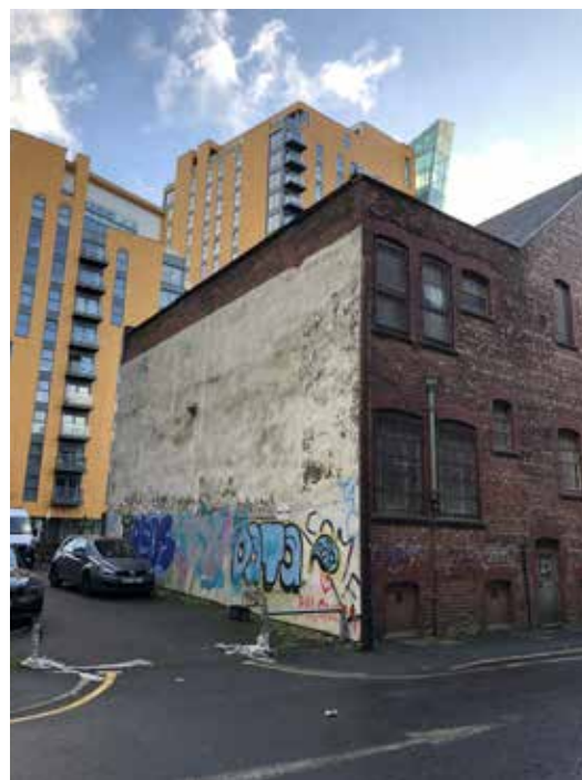
Side elevation (east), corner with Rear Elevation
