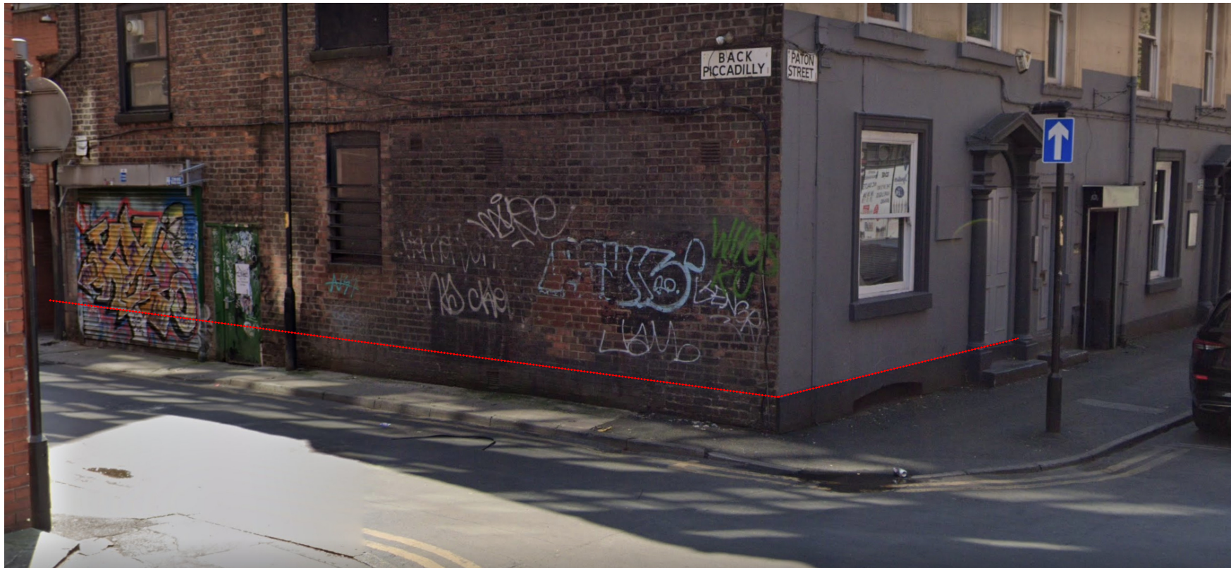
The red line indicates the internal floor level.
