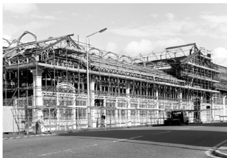
City Hall at the corner of Liverpool Road & Lower Byrom Street during remedial & re-purpose works to turn it into the Manchester Air & Space Museum in 1981. Note the complete removal of roof and elevation coverings.
