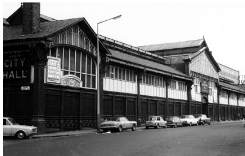
City Hall at the corner of Liverpool Road & Lower Byrom Street in 1972. Note the chimney to the west gable, now demolished.
