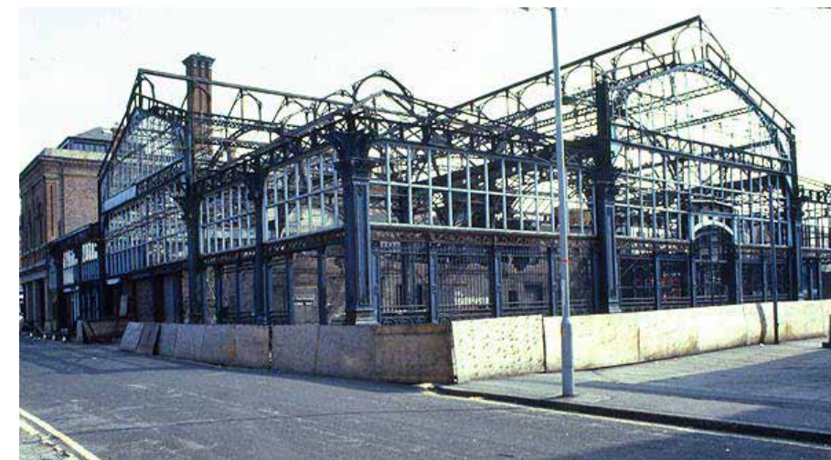
Upper Campfield circa 1980s possibly during remedial works to the facade and structure as the ones to Lower Campfield.
