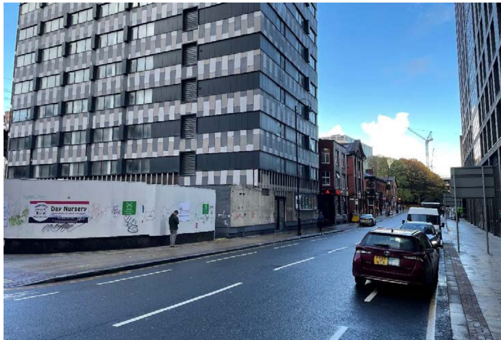
Figure 4.3: View north-east along Charles Street and towards Lass O' Gowrie Public House from junction with York Street
