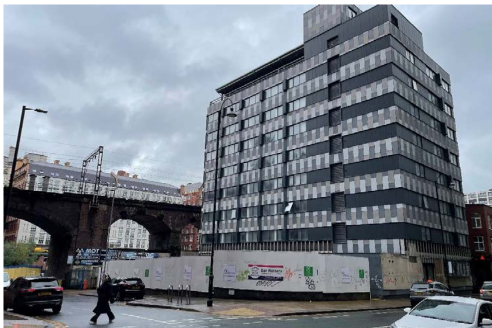
Figure 4.1: View through the Site towards MSJAR Viaduct and India House from Charles Street
