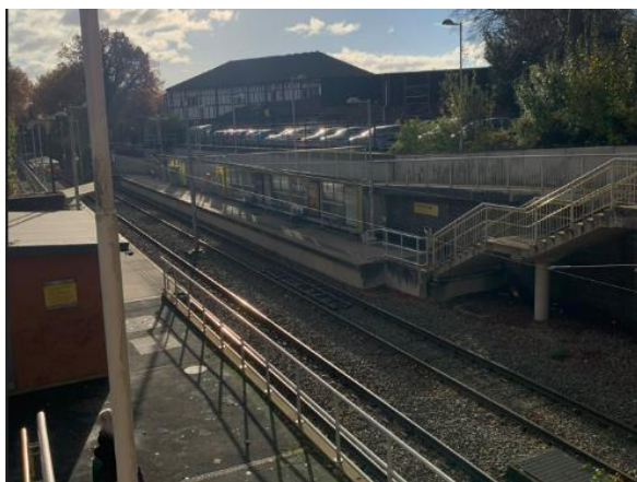
Photograph 15: West Didsbury Tram Stop
