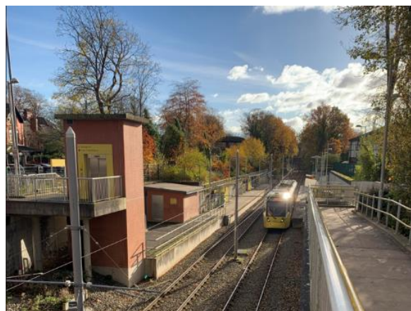
Photograph 16: West Didsbury Tram Stop
