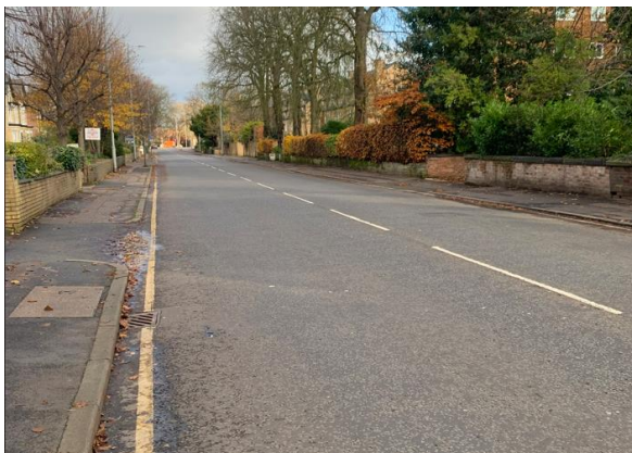
Photograph 5: Palatine Road Existing Conditions Facing North
