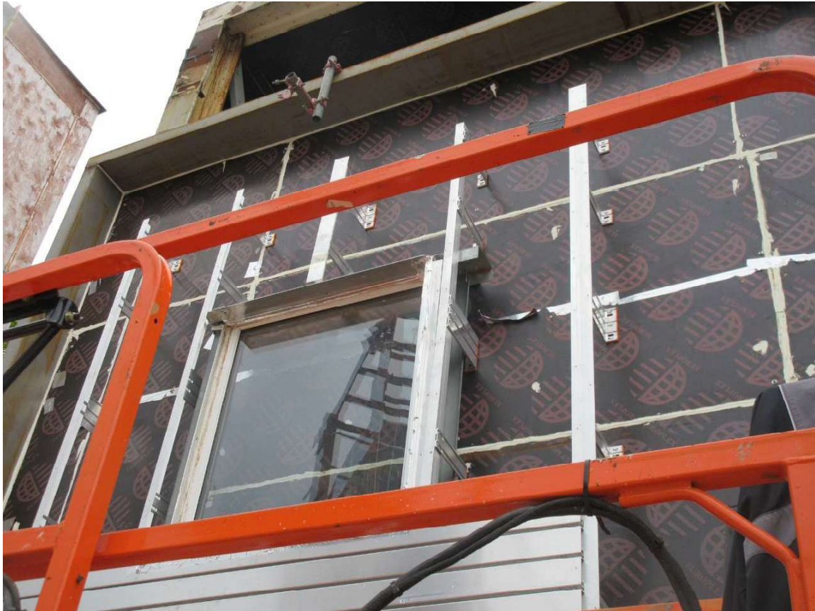
TEST SAMPLE DURING DISMANTLE
