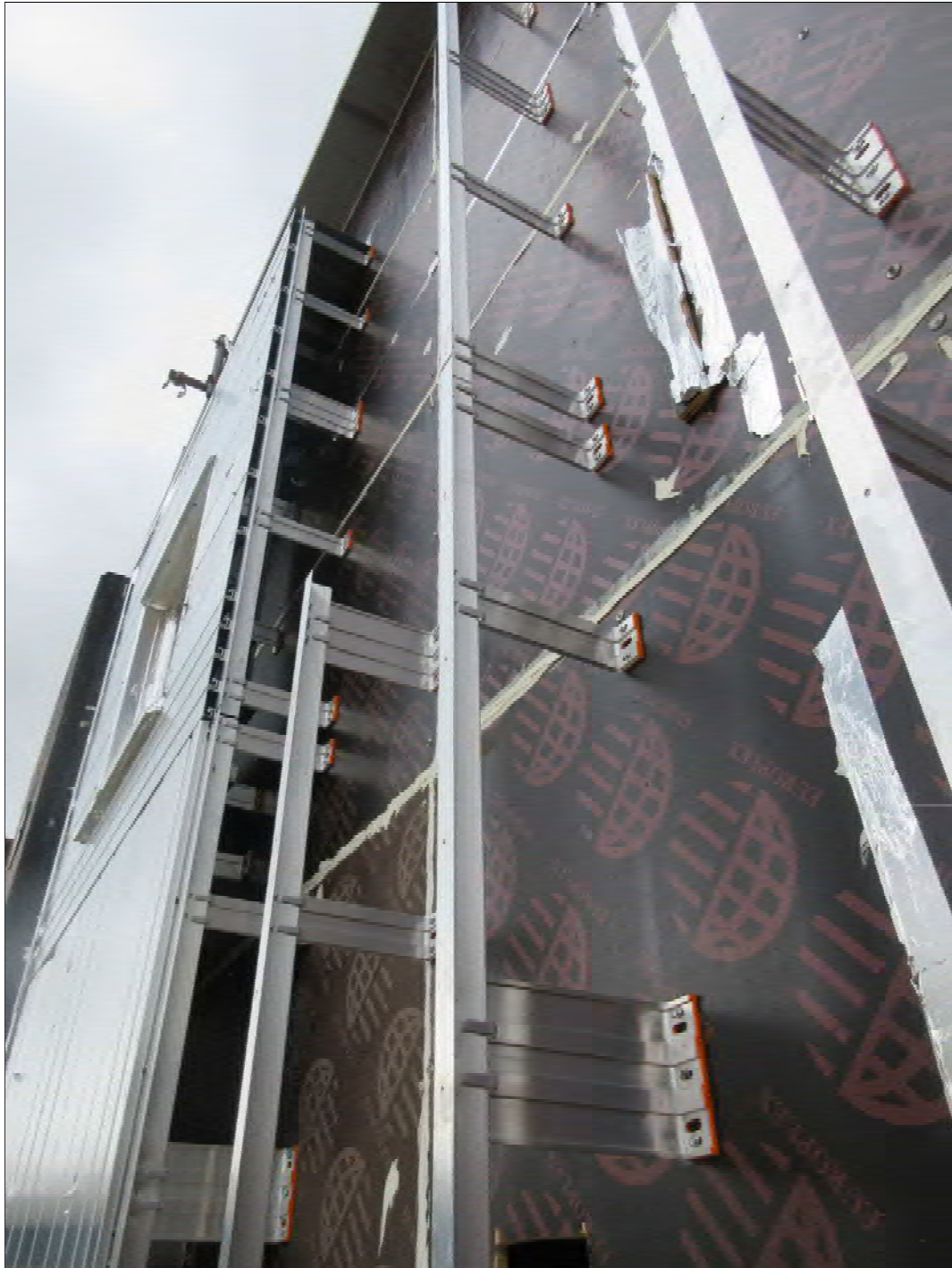
TEST SAMPLE DURING DISMANTLE
