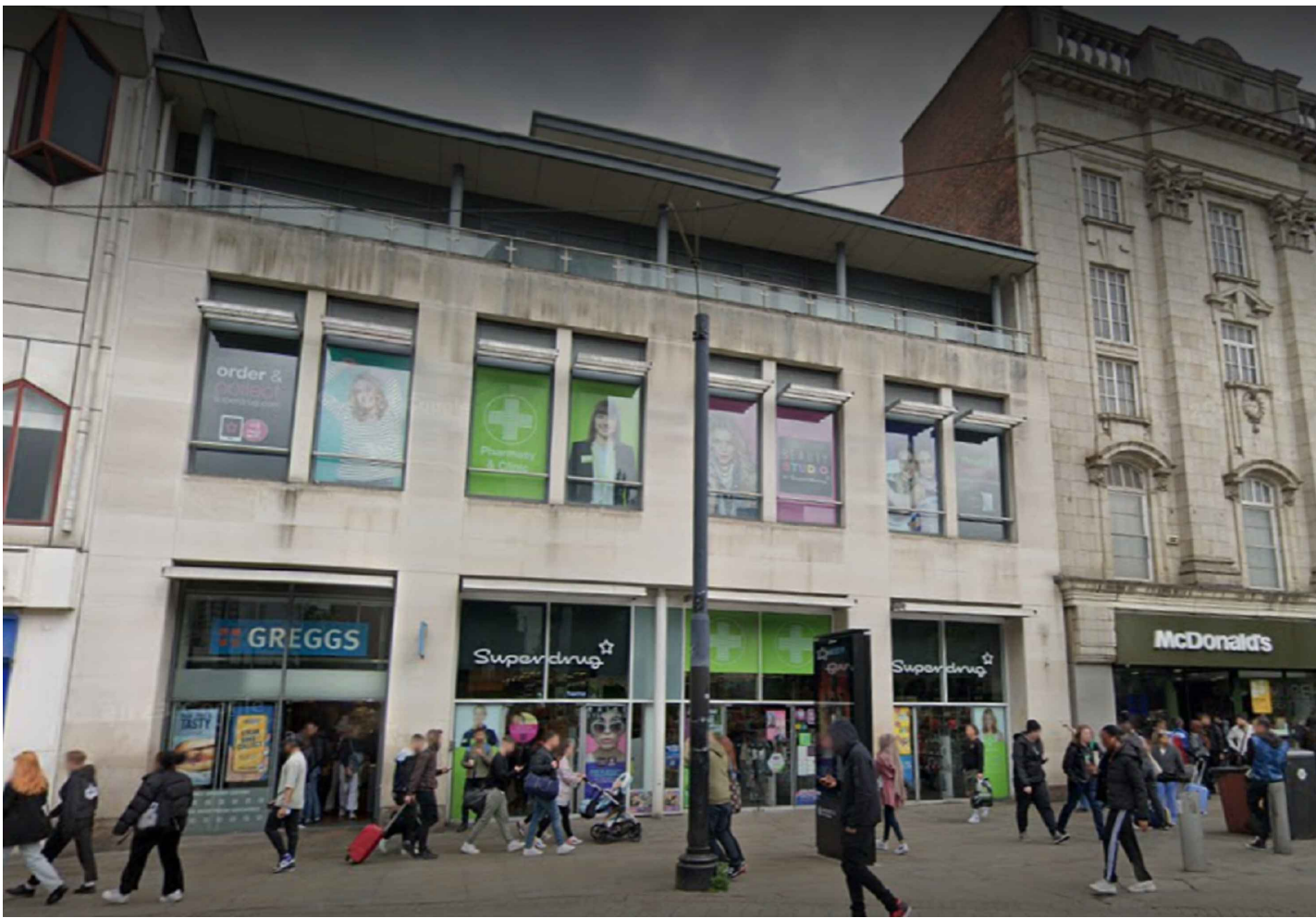
Existing Fascia NTS
