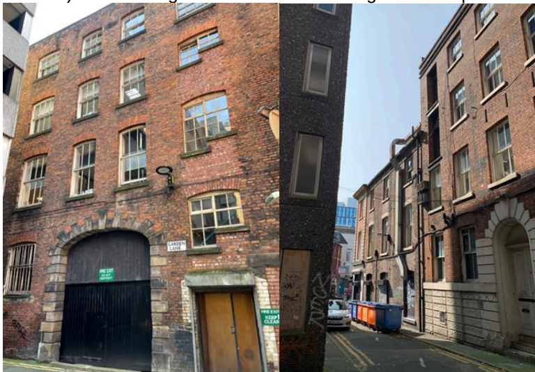
Photos o) and p) The carriage workshop and the warehouse
