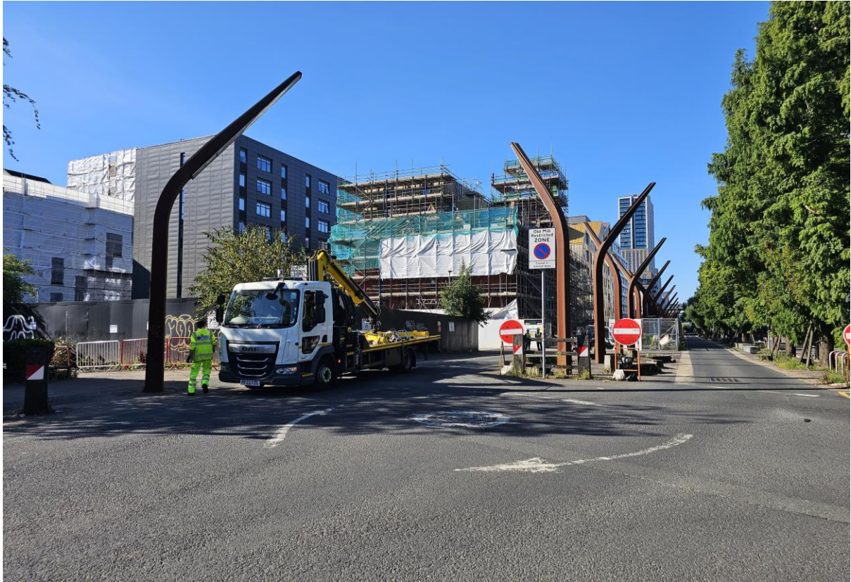
Plate 8: Photograph taken south-west from Old Mill Street facing the Site, hospital and modern buildings.
