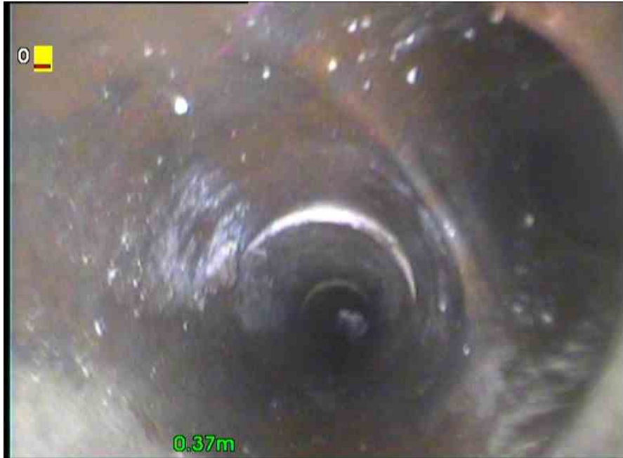
, 00:00:20, 0.37 m Junction at 2 o'clock, diameter: 100mm
