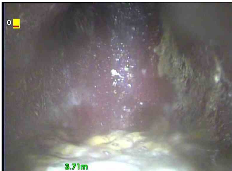
, 00:01:35, 3.71 m Finish node type, major connection without manhole, reference number: SVP, Soil Vent Pipe
