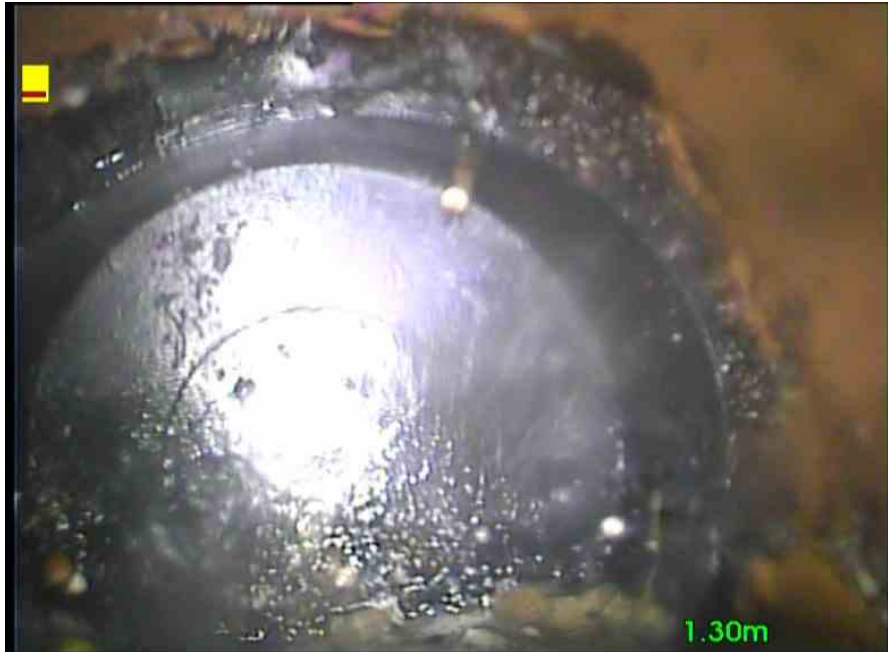
, 00:00:36, 1.30 m Finish node type, gully, reference number: Swg, surface water gully
