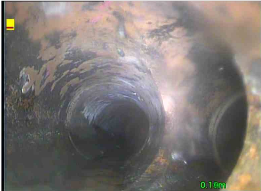
, 00:00:14, 0.19 m Junction at 3 o'clock, diameter: 100mm
