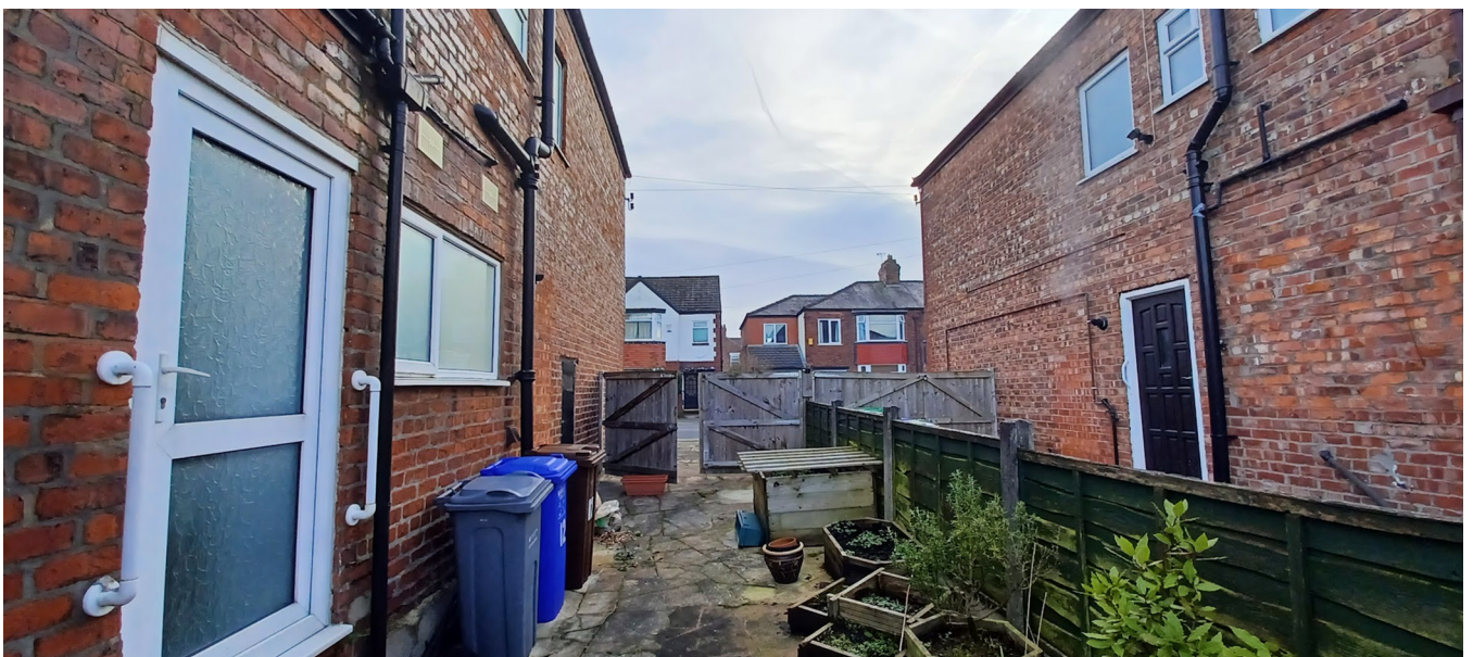
Figure 4. View along side of property.
