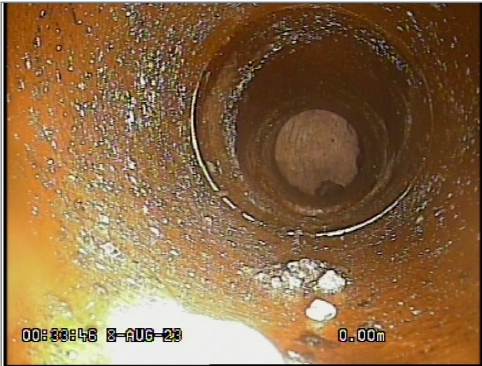
Start node type, manhole, reference 6602
