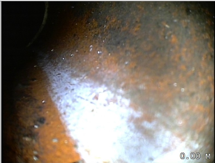
Start node type, manhole, reference MH6
