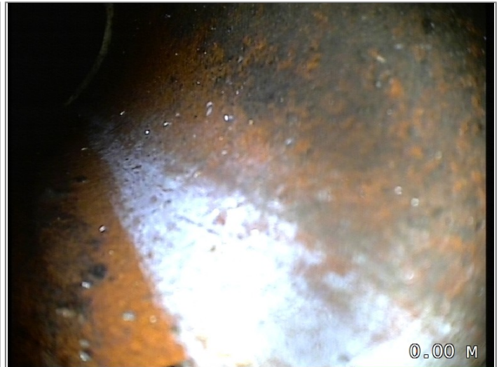
Water level 5% height/diameter
