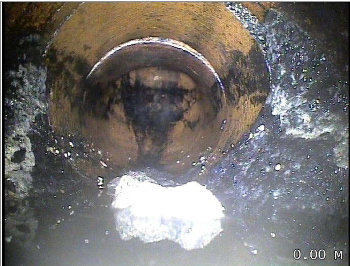
Start node type, manhole, reference MH1
