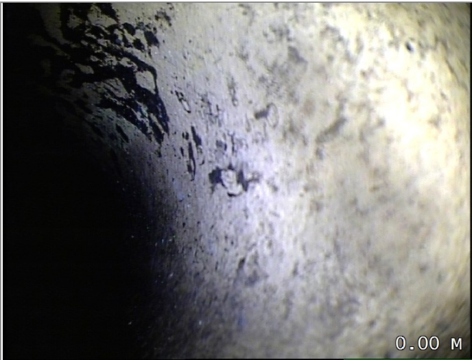
Start node type, manhole, reference MH6
