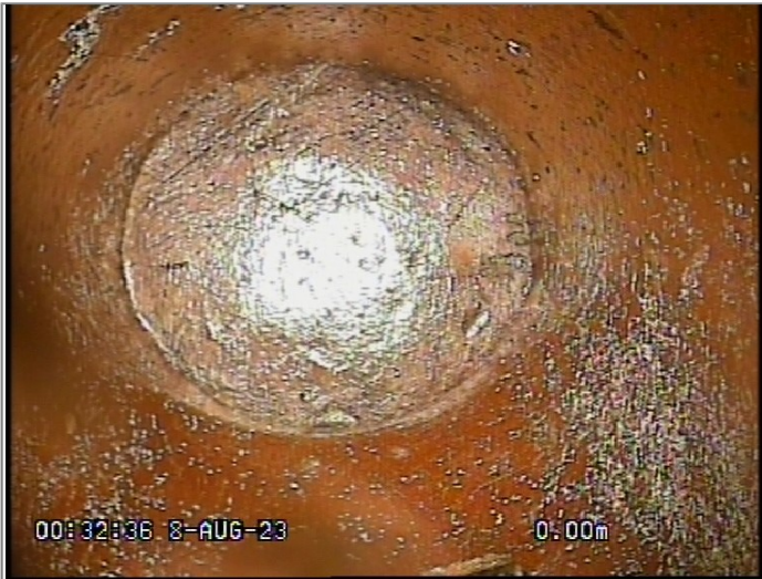
Start node type, manhole, reference 6602
