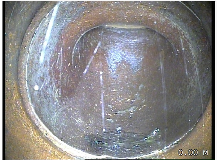
Water level 5% height/diameter
