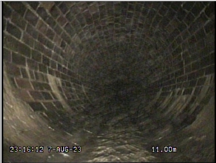
Start node type, manhole, reference 7600
