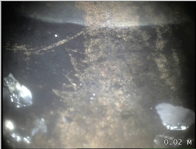
Start node type, manhole, reference MH1
