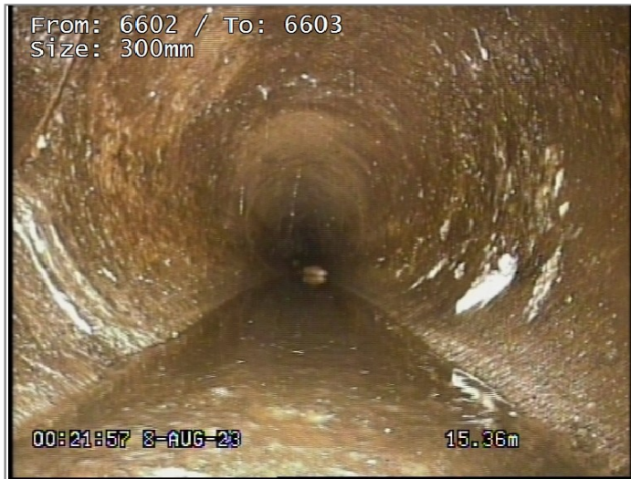
Connection other than junction at 10 o'clock, diameter 150mm
