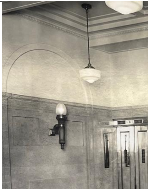
Figure 9: Ground floor Entrance Hall – two lifts originally arranged either side of the staircase. Close up image also provide detail of the brass, wall mounted lighting and pedament lighting which historically featured within these principal spaces. The walls featured recessed arch detail with exposed stone. Source: Manchester Archives Manchester Archives
