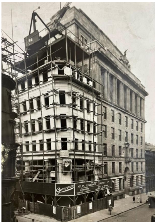
Figure 11: Atlas Chambers under construction Source: Manchester Archives
