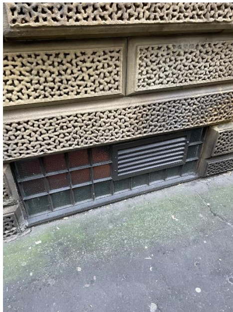
Figure 27: External view of Lombard Chambers basement light, shown to be altered with modern vent unit.
