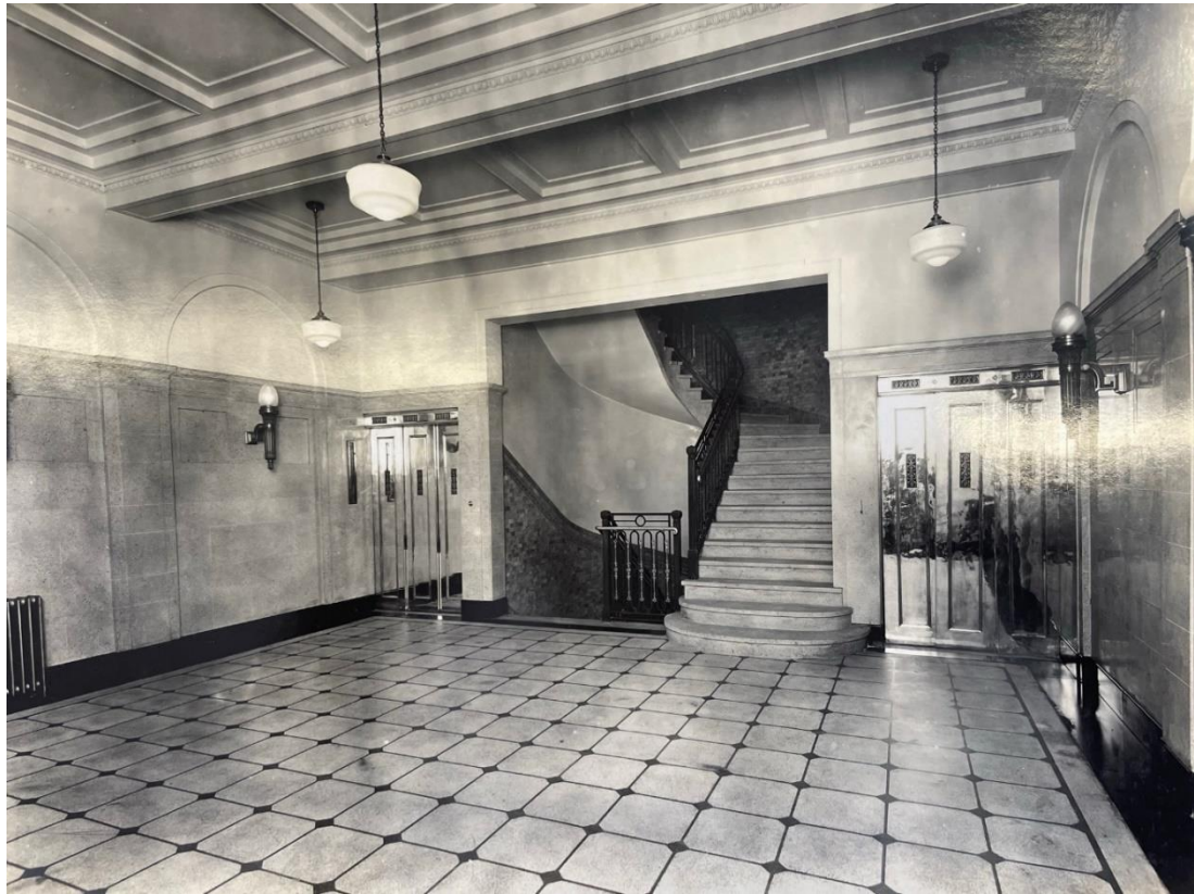
Figure 8: Ground floor Entrance Hall – two lifts originally arranged either side of the staircase. The historic image provides greater understanding of the historic character of the entrance hall, principally the design of the floor tiles and detail of the coffered ceiling. Source: Manchester Archives
