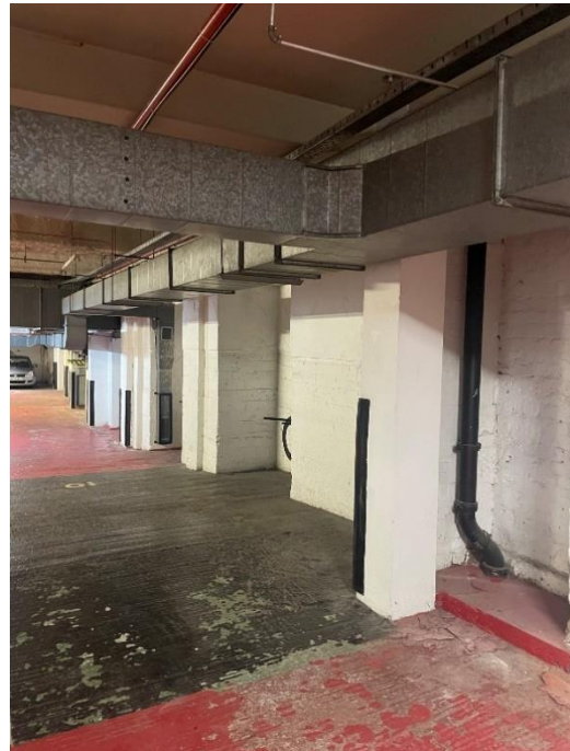
Figure 26b: Basement area, under Lombard Chambers. Stripped out with some original brick external walls (overpainted white).
