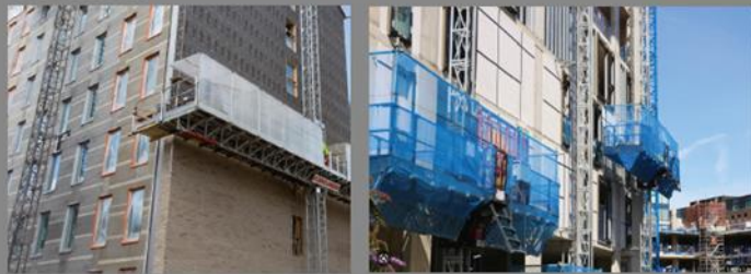
Typical mast climber protection netting to protect against material falling onto waterway
