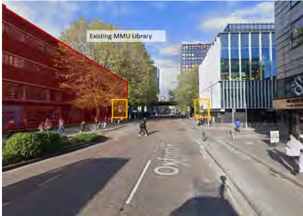
Figure 4 View from Traffic light 2 travelling north, existing building
