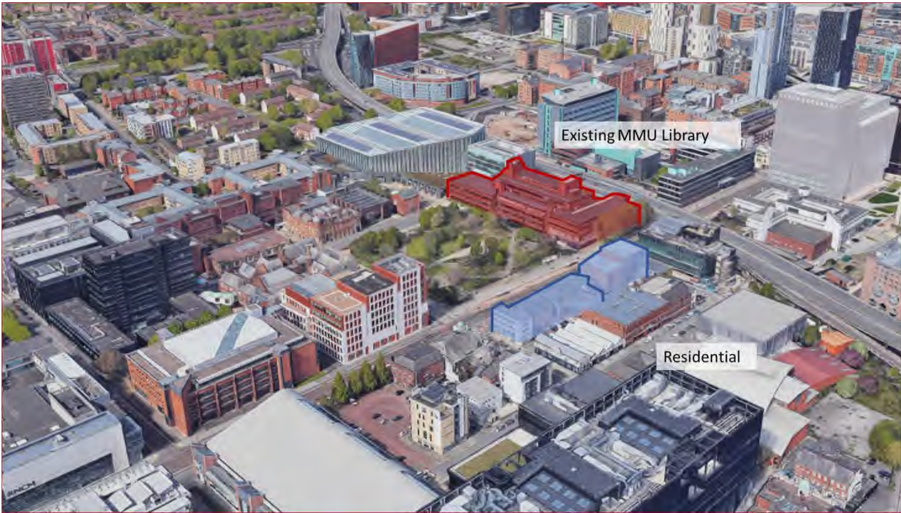
Figure 3-2 Buildings sensitive to the new MMU Library development
