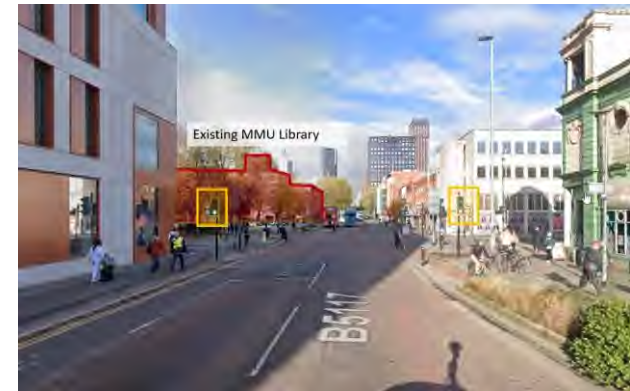
Figure 2 View from Traffic light 1 travelling North, existing building
