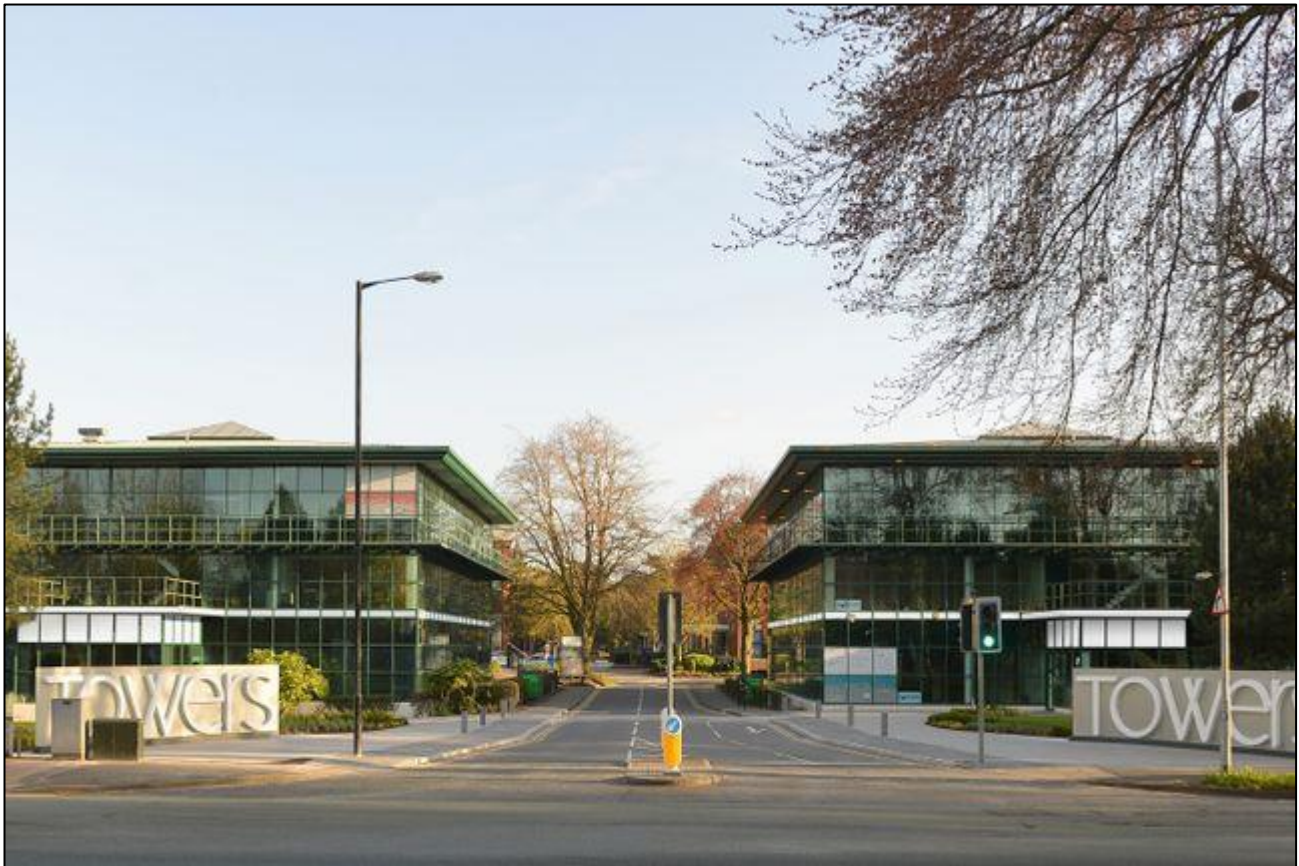
Figure 1. Entrance from Wilmslow Road
