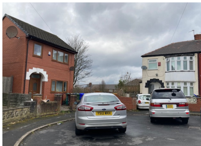
View of the frontage from Enfield Drive
