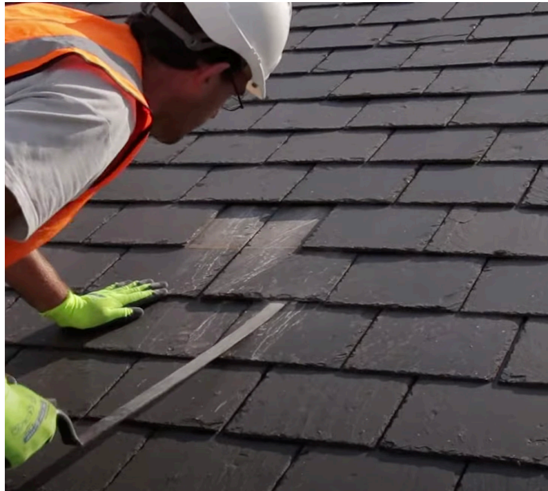
Existing slate tiles are carefully removed and stored for future use.
