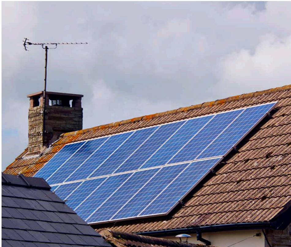
Good example of low profile supporting frame
