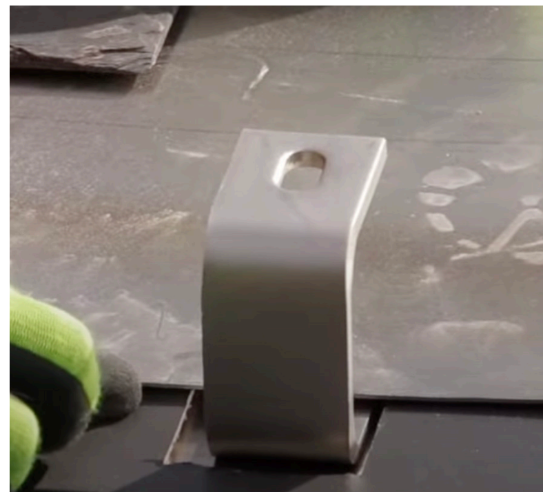
New reclaimed slate roof tile is cut to form a slot for the anchor and another layer of lead flashing is installed to keep the roof watertight
