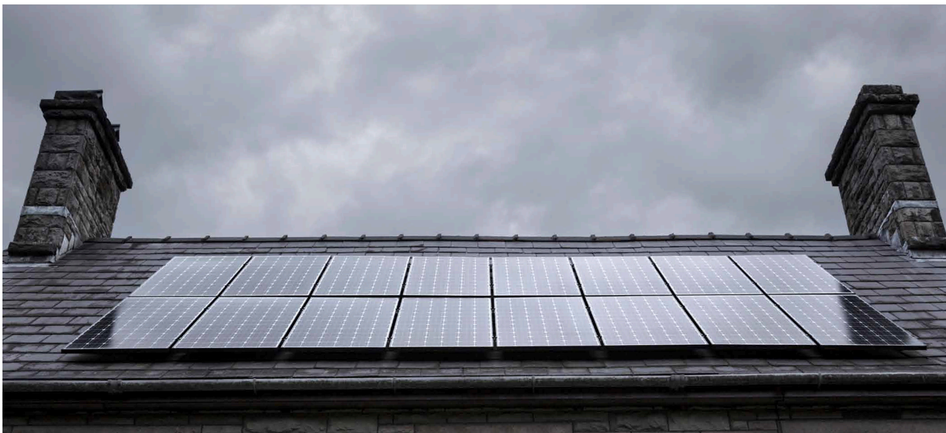
Good example of how the panels arranged symmetrically and evenly between chimneys, ridge and eaves
