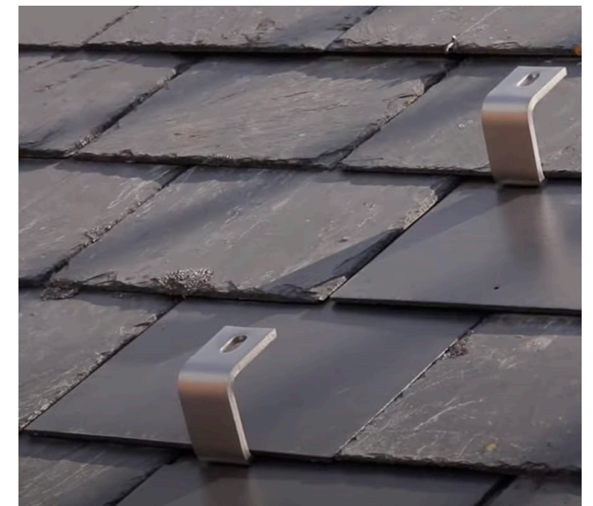
New roof tiles blend in with existing tile with no original slate tiles damaged. Please note proposed anchors will be anodised black.
