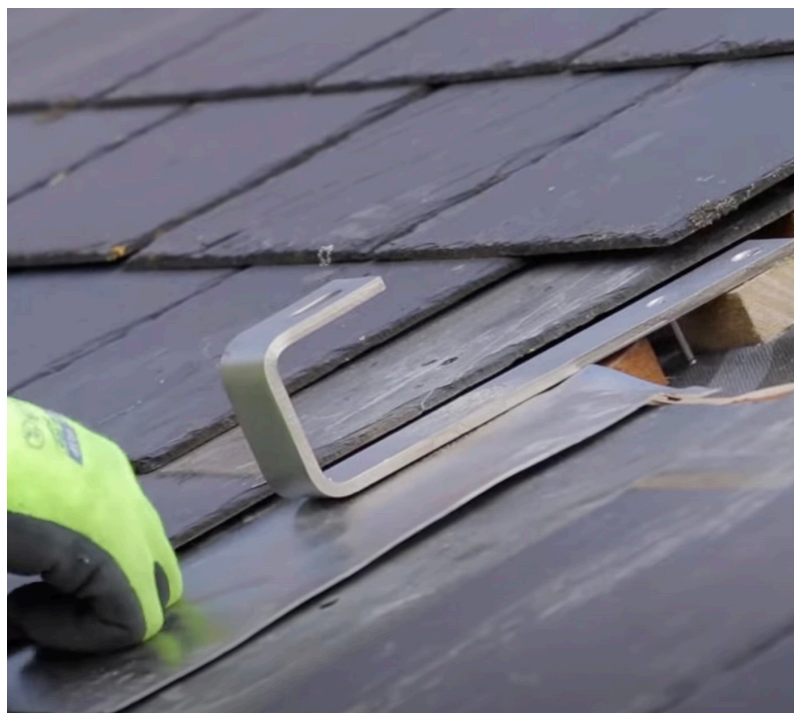
Lead flashing installed over existing roof tiles.
