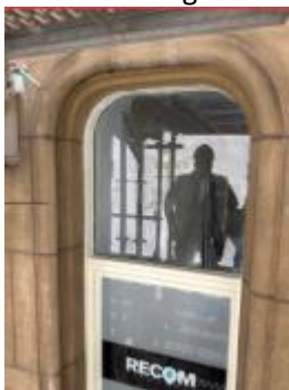
01-05-GE3 – 1no 675 x 725 with shaped top, currently clear glass, will need a leaded light manufacturing to match - 01-05-GE1 – 1no 675 x 715 with shaped top
