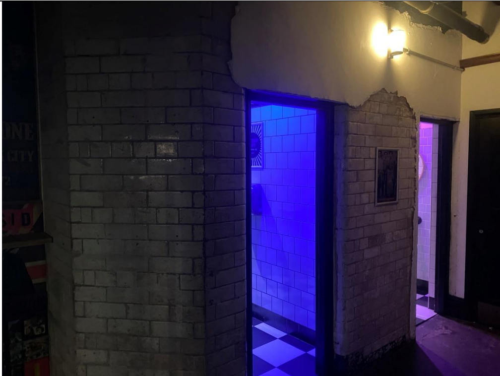
Figure 34: Basement, looking north across space towards modern W.C.s. Original white glazed brick features. All W.C. fixtures and fittings are modern and of no heritage significance.
