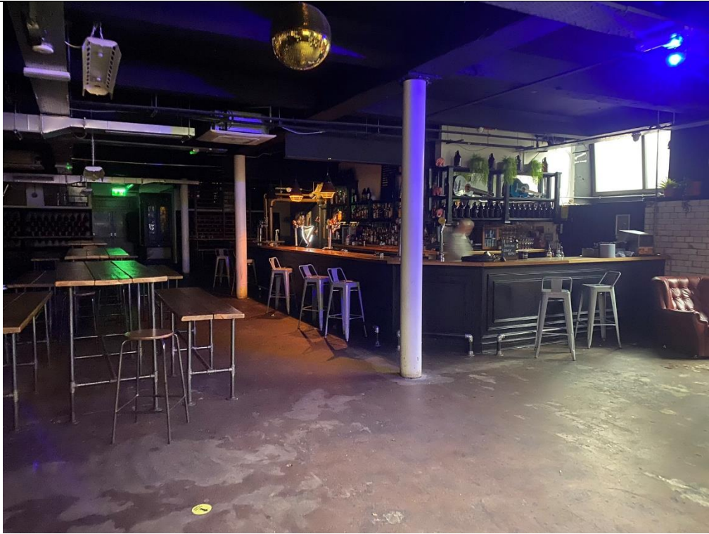
Figure 32: Basement, looking south-east across space. Original exposed columns and concrete floor. Modern bar and associated bar fittings (including M&E / lighting) have been inserted. Original white glazed brick is apparent to basement walls.
