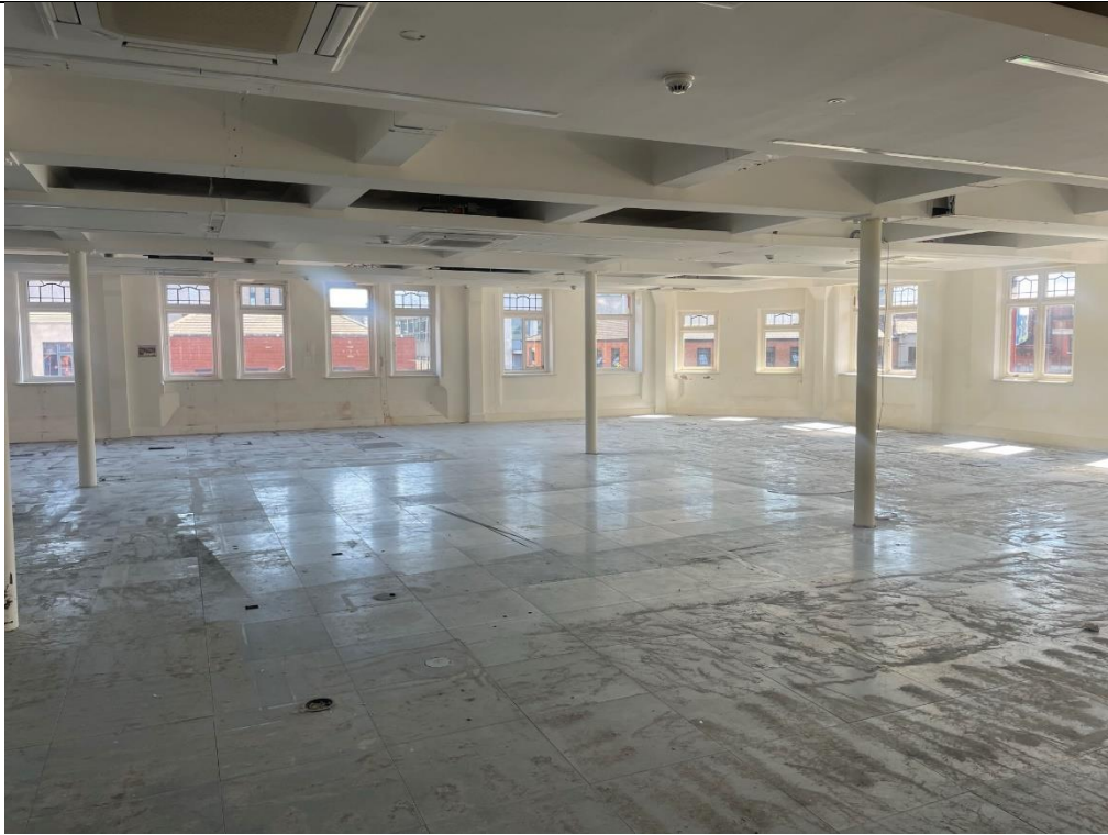
Figure 43: First Floor. Looking south-west across open floorplate. Original column structure, ceiling grid and windows. Modern floor tile.
