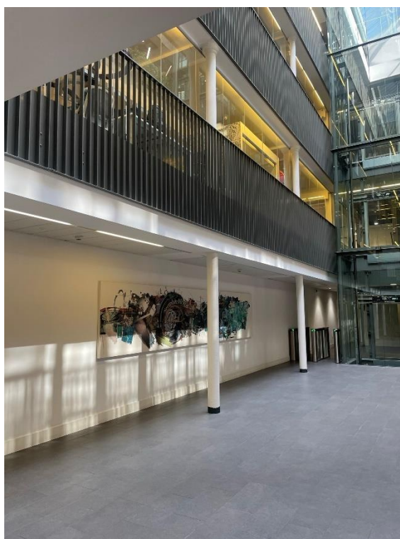
Figure 39: Reception / lobby space. Looking north-west. Modern wall inserted to ground floor to create a separate unit. Glazing features to levels above.
