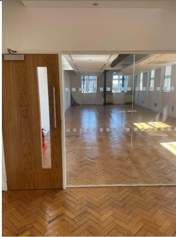
Figure 51: Fifth floor. Example of modern alteration to fifth floor to create office unit Modern glazing, doors and bulkheads. Original parquet flooring features / exposed throughout the space.
