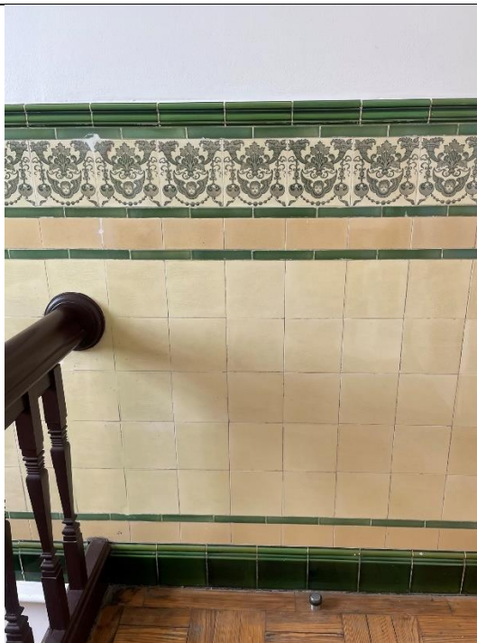
Figure 50: Fifth floor, stairwell. Original cream and green glazed tiling feature to principal areas on fifth floor.
