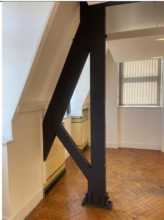
Figure 52: Fifth floor. Example of original supporting truss, exposed within space. Modern dropped ceiling.
