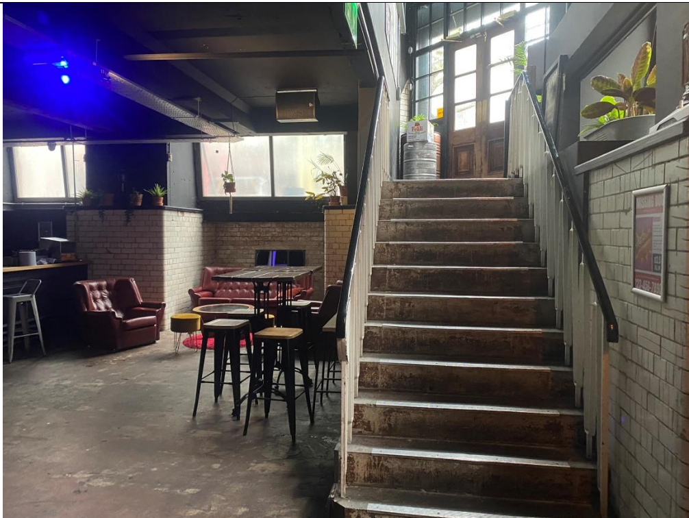
Figure 31: Basement, west corner. Modern stair inserted, leading up to street level (Dale Street / Spear Street corner). Original white glazed brick is apparent to basement walls. Original concrete floor is also exposed.
