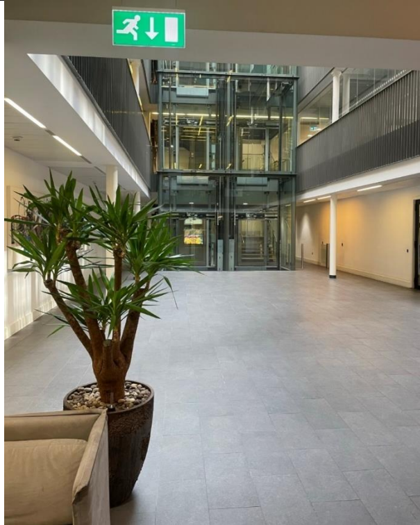
Figure 36: Reception / lobby space. Modern floor tiles, glazed lift core and wrap-around balconies feature. Original column layout is discernible. The space did originally feature a central lightwell, as evidenced within the early 1900s plans.
