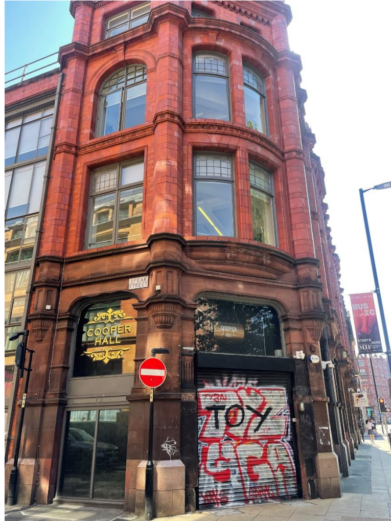
Figure 29: Dale Street / Spear Street corner. Ground floor entrance, with roller shutter door leading into basement area / former nightclub. Entrance and windows shown to have been altered under previous Planning and LBC consent.
