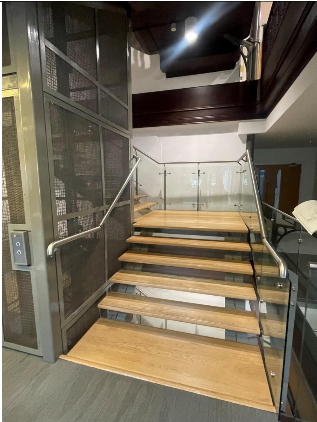
Figure 42: Main stairwell. Modern stair and glazed balustrading up to third floor level. Early 20th century lift structure features to centre of main stairwell.
