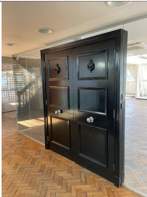
Figure 48: Fourth floor. Original parquet flooring. Modern glazing to create open effect office units. Replacement door.
