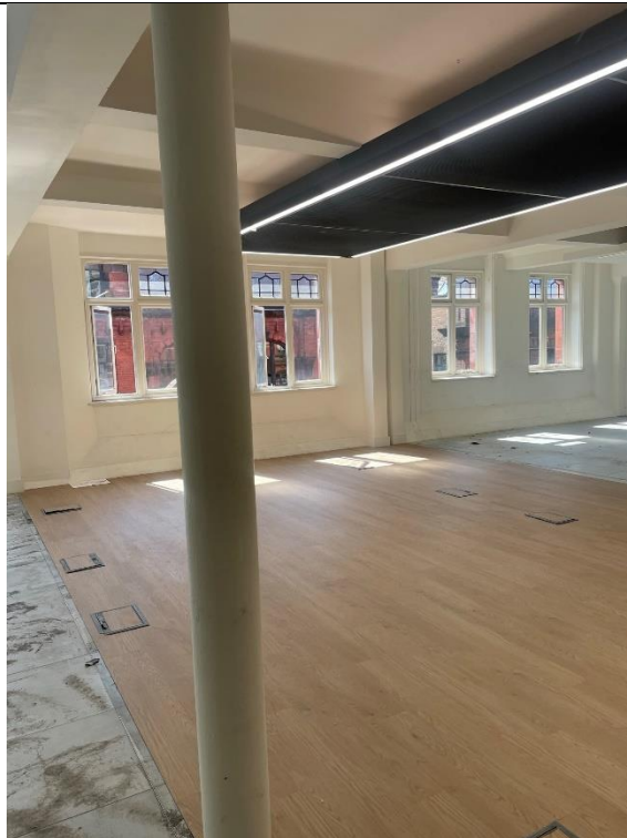
Figure 44: First Floor. Looking west across open floorplate. Original column structure, ceiling grid and windows. Modern floor sample (timber effect) features. Modern M&E sample features.
