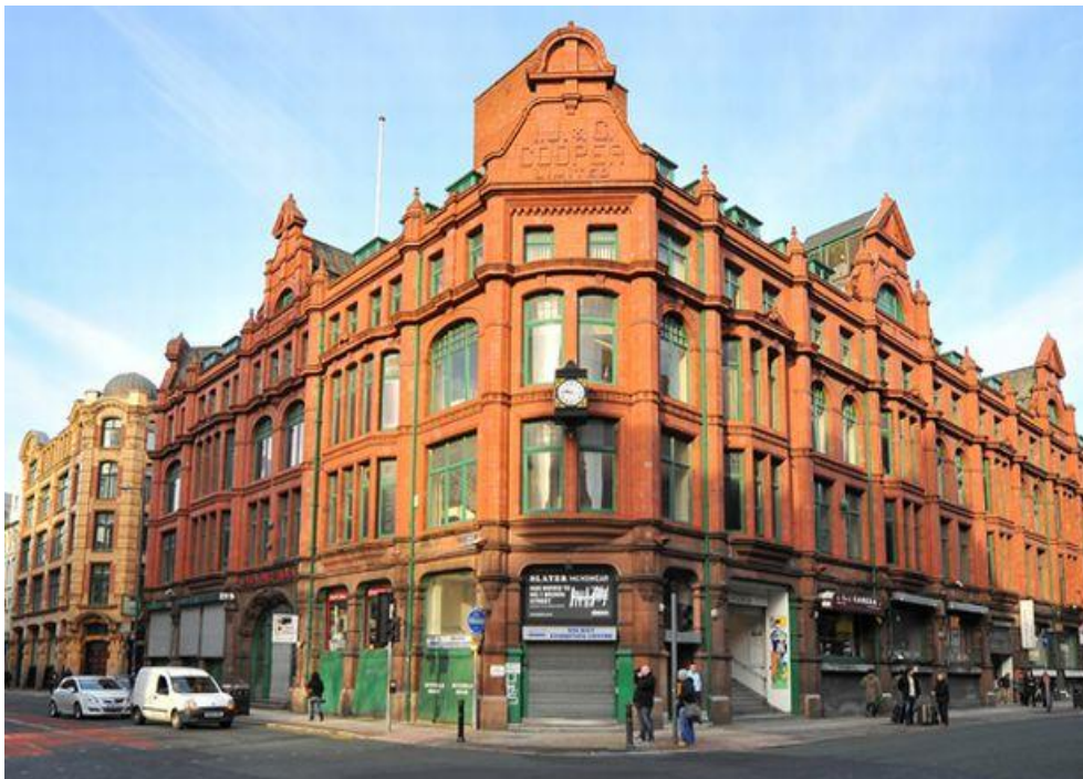
Figure 1: Sevendale House (Grade II), as viewed from Stevenson Square, looking north-west. Source: Google Images, Manchester Evening News article. September 2014.
