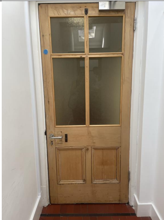
Figure 54: Fifth floor. Original early-20 th century door leading from corridor into kitchen area. One of the few remaining original doors throughout the building.
