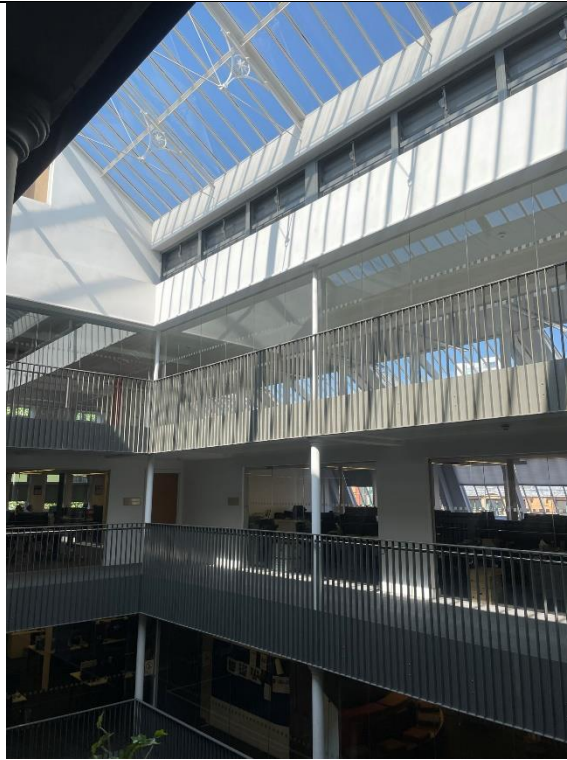
Figure 47: Central lightwell. View looking west. Modern balustrading and glazing to form individual office units.
