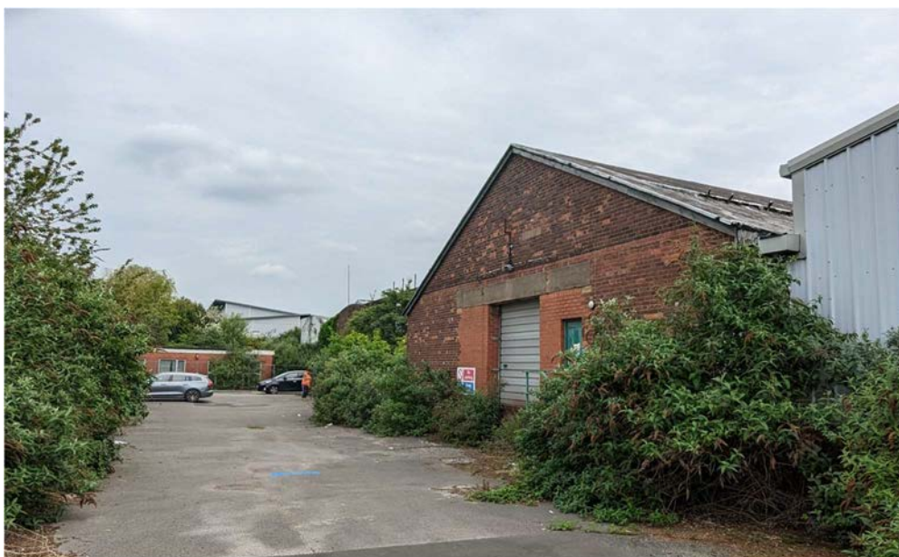
Figure 2.2 - Photograph of the area of hardstanding to the front and west of the building.
