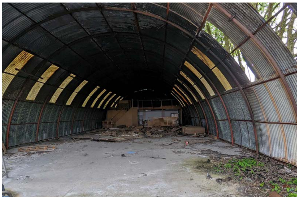
Figure 2.3 - Photograph of the prefabricated building in the eastern part of the site.
