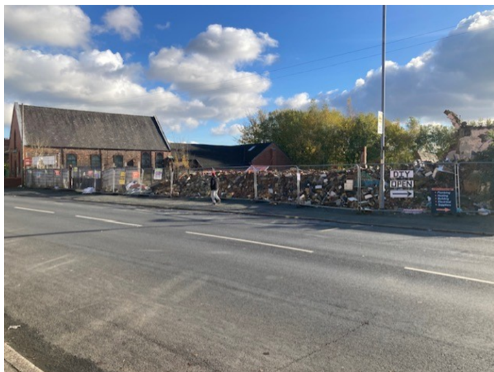
View of the application site from Kenyon Lane
