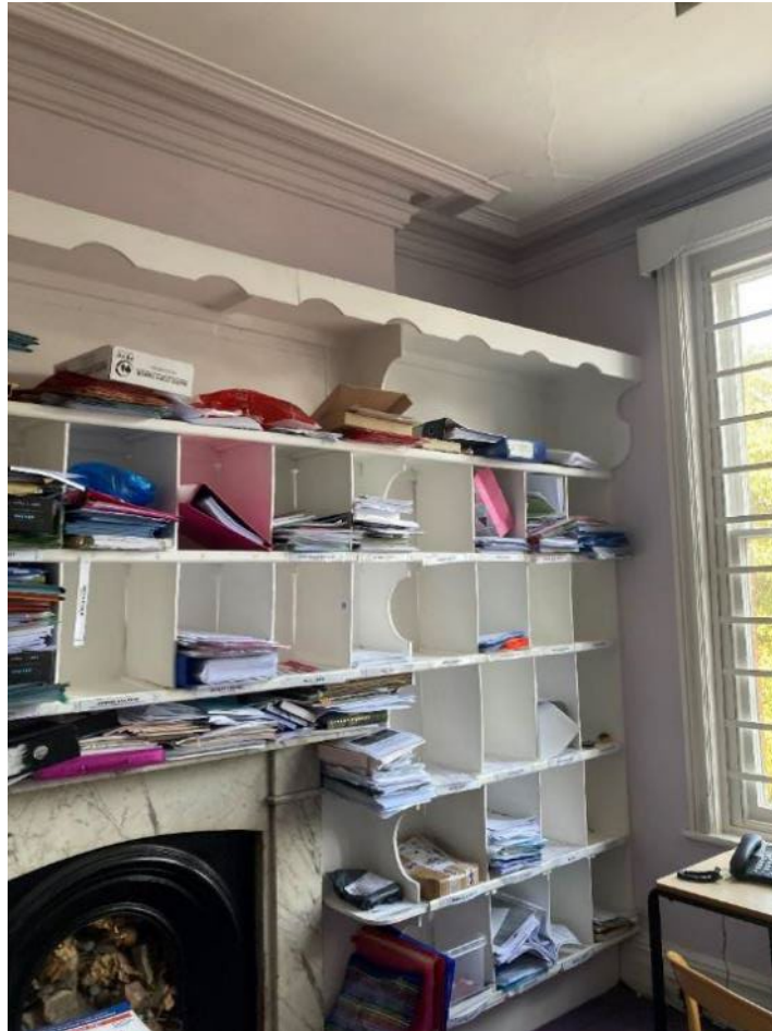
Plate 7. Original fireplaces, ceiling coving and windows amongst modern school fittings
