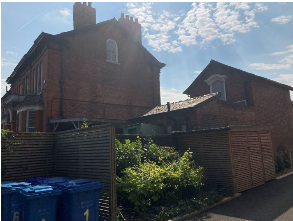
Plate 2. View of the west facing elevation of the main building and original outbuilding
