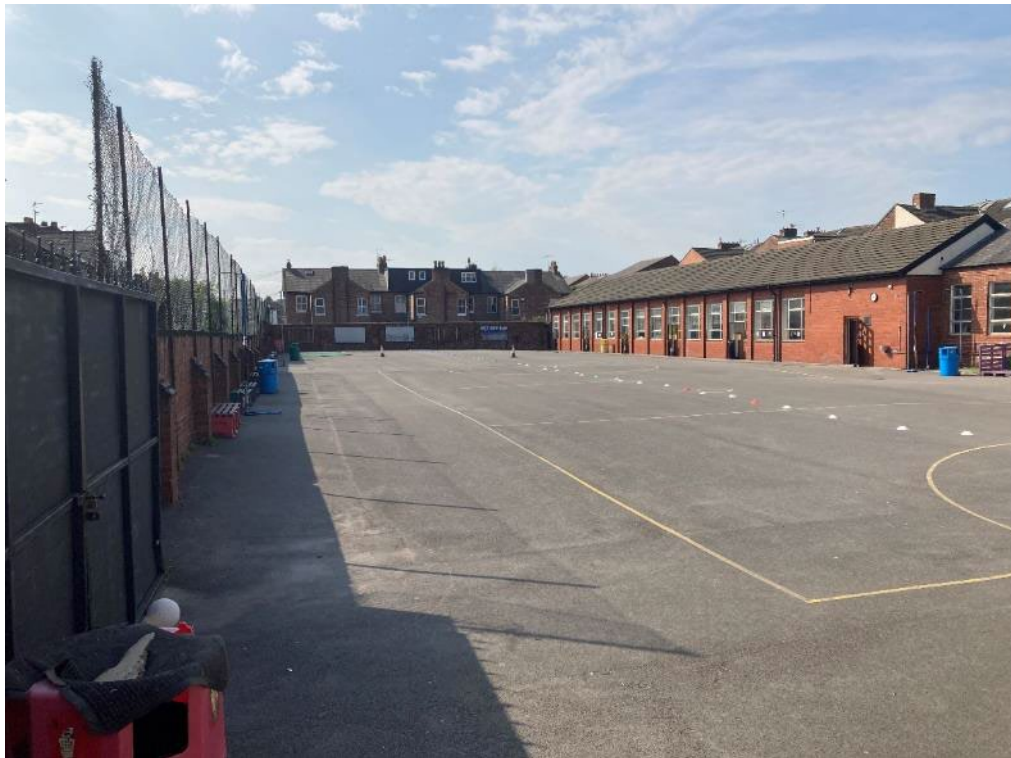
Plate 14. South facing view of the playground and extent of the site
