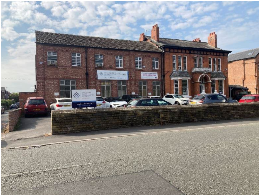
Plate 1. View of north facing principal elevation. The former Carlton House is on the right with the east convent extension on the left
