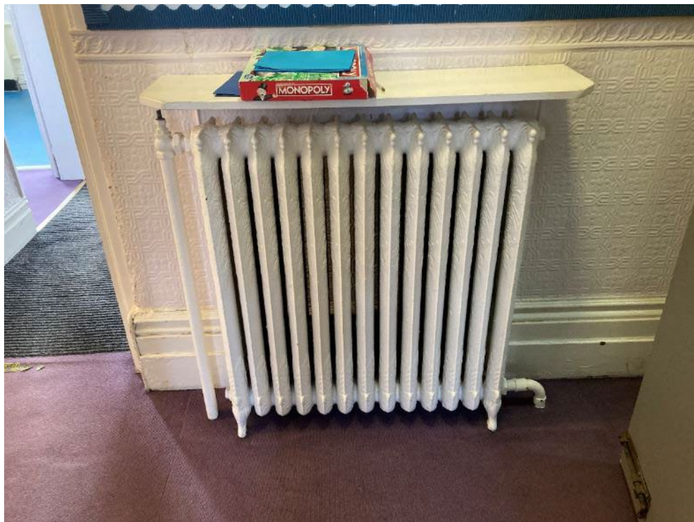
Plate 6. Cast iron radiator within the main entrance hall
