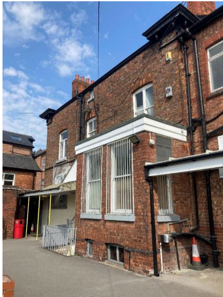
Plate 10. Rear elevation of the original Carlton House
