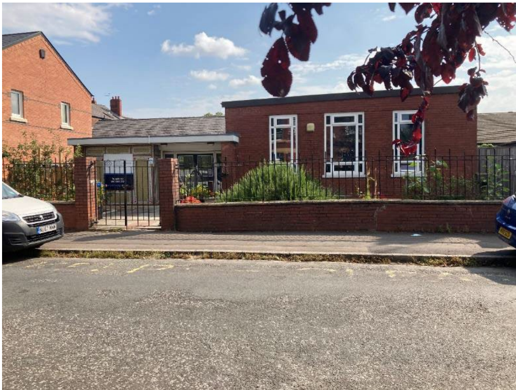
Plate 4. View of western extension to the school onto Stockton Road
