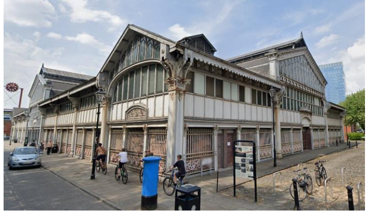
Figure 96: The south elevation (left) and east elevation (right) (2018)
