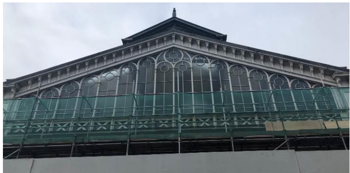
Figure 94: The central glazed Venetian windows to the east elevation. (2023)
