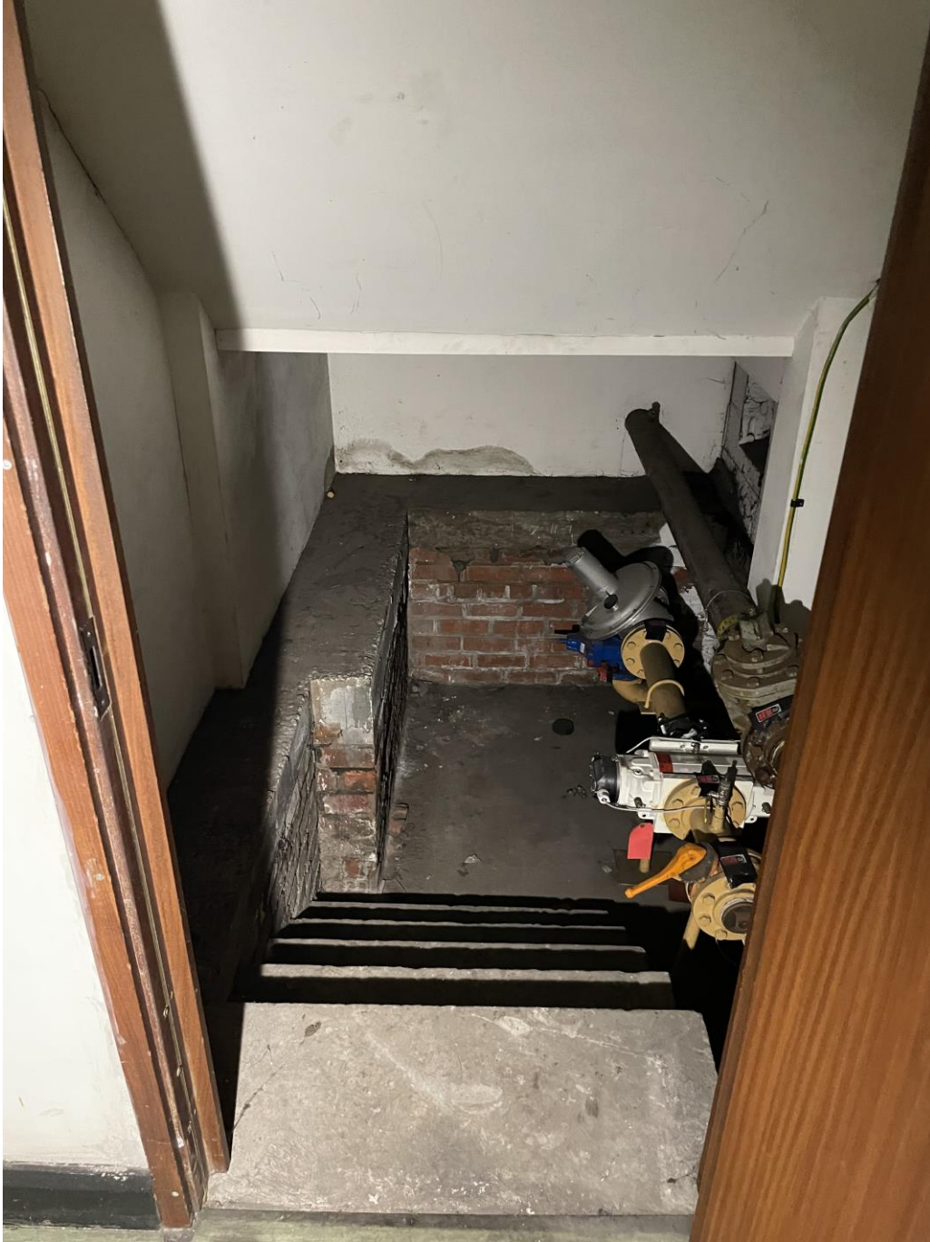
Figure 116: Looking down into a lower level utility space within the south-east stairs.
