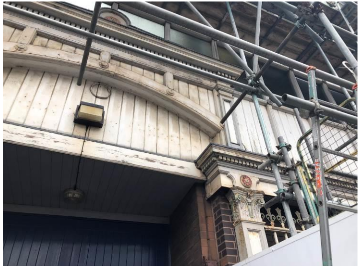
Figure 95: The lower parts of the west elevation. (2023)
