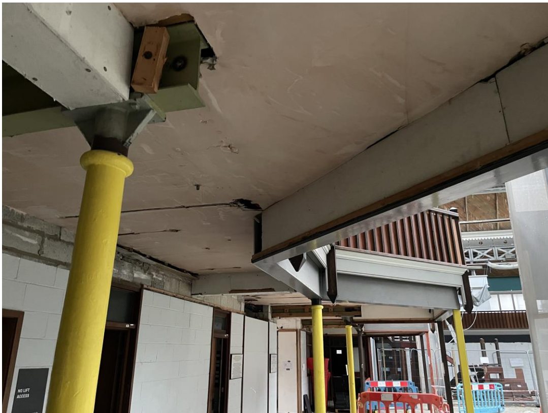
Figure 109: Detail of the heads of one of the existing columns to the eastern side of the building.
