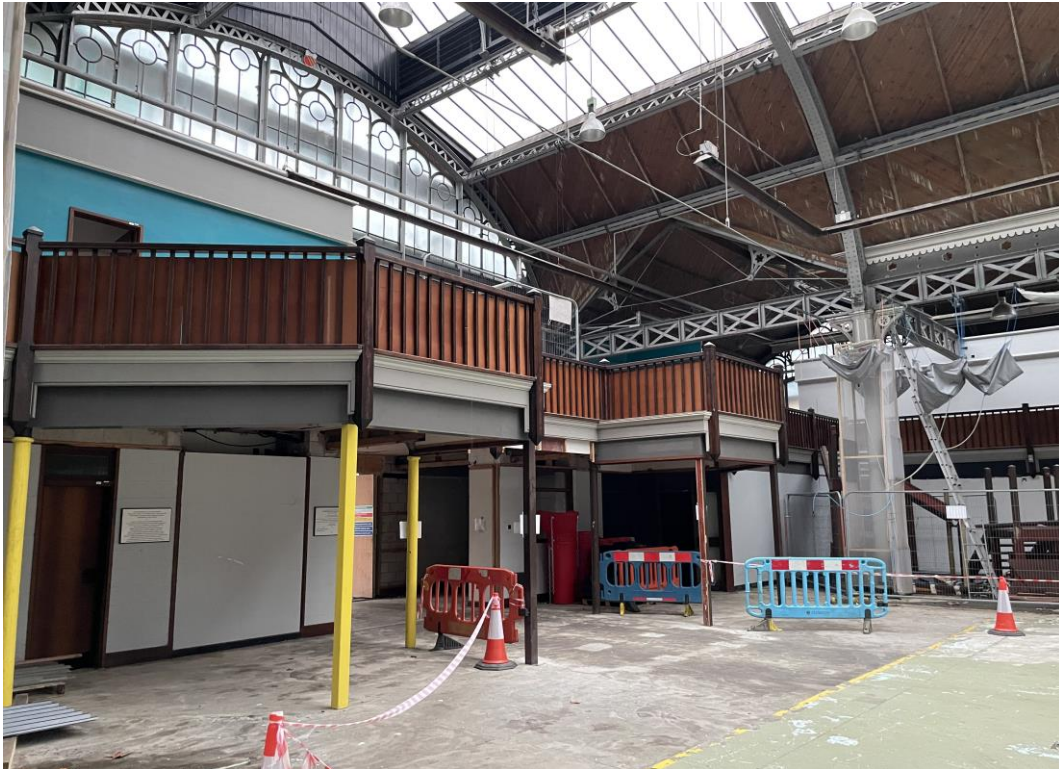
Figure 106: Looking south-east towards the eastern end of the building, showing the modern 1980s extended balcony.
