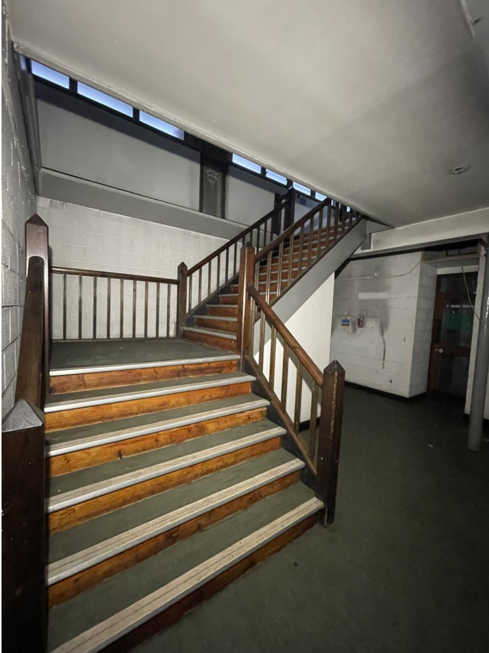
Figure 114: Looking south into the south-east staircase.
