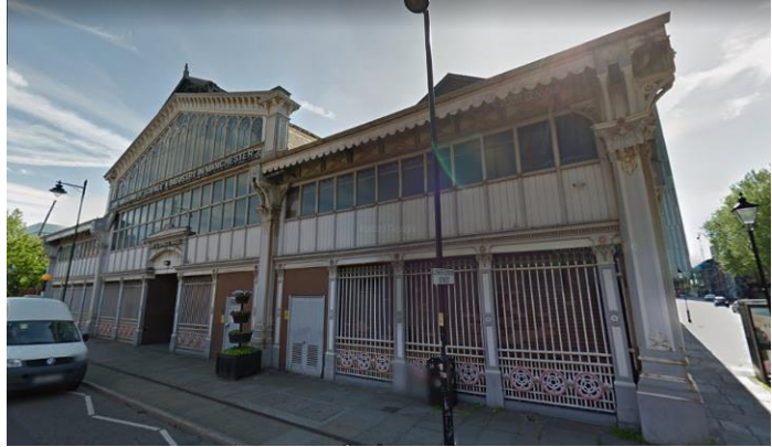
Figure 93: The southern elevation as seen from Lower Byrom Street. (2018)
