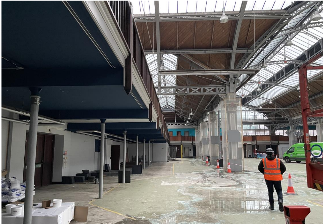
Figure 102: Looking east along the north balcony from the western end.
