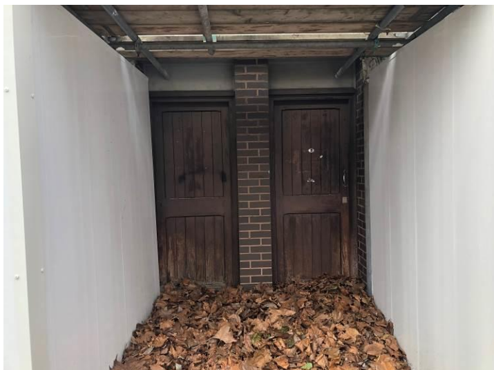
Figure 98: Examples of 1980-3 doors to the east elevation. (2023)
