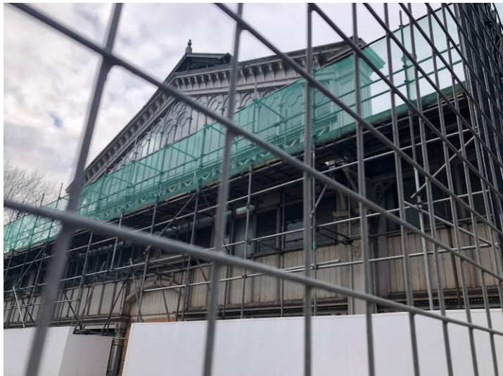
Figure 97: The east elevation. (2023)
