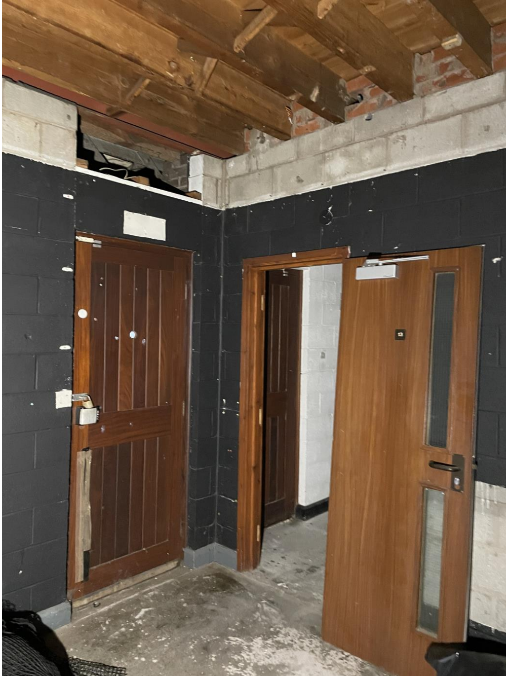
Figure 113: Looking south-east into the corner of the building showing the 1980s breeze block room partitions.
