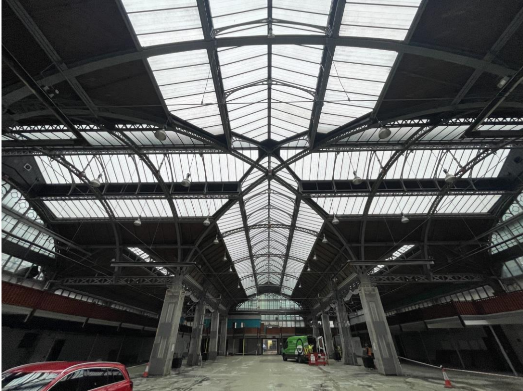
Figure 122: Looking up at the roof.
