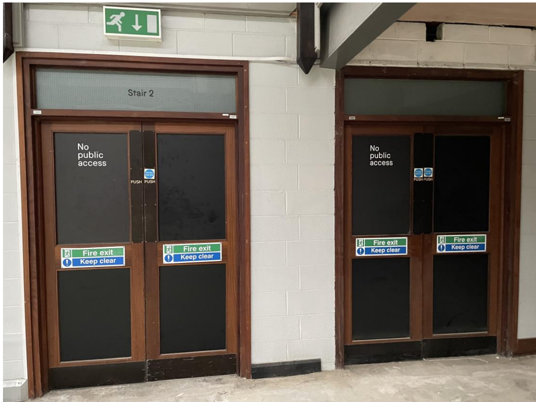
Figure 108: Two pairs of early 1980s doors to the north-east corner.
