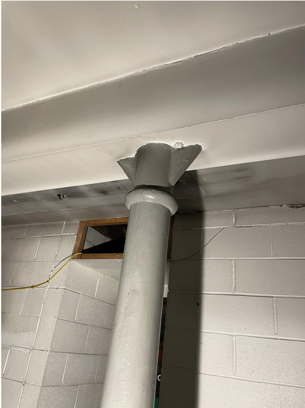
Figure 115: Detail of an earlier column in the south-east staircase hall.
