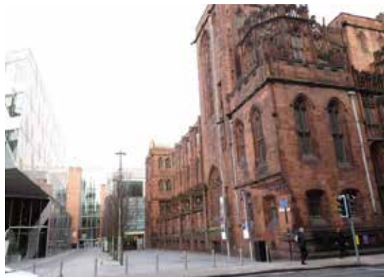
Fig. 11 View west along Spinningfields showing The Avenue, left, and the Magistrates' Court beyond
