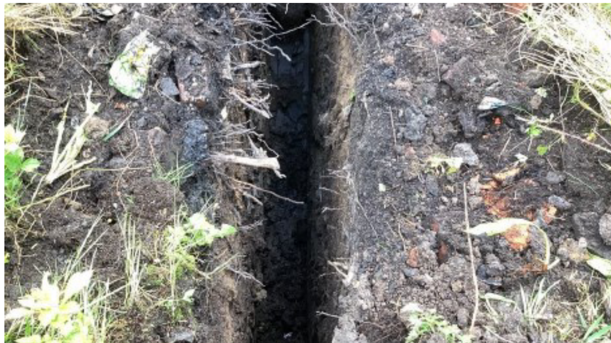
TP03: South side of the trial pit.
