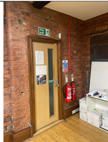
Figure 17: Example of modern door proposed to be upgraded. Skirting boards in these spaces are all modern and of no heritage significance.
