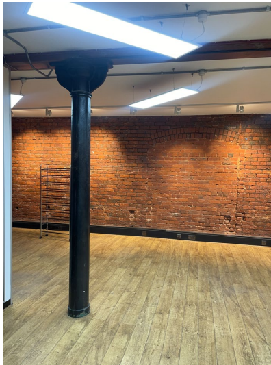
Figure 8: Looking north east across space (former berghaus unit, 3 rd Floor). Illustrating original columns and redbrick walls of high significance. Flooring is modern overcovering original floor below.
