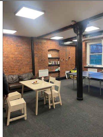
Figure 13: Looking east within north unit, illustrating original brick wall and column arrangement. Modern plasterboard ceilings, lighting and carpet overcovering original floor.
