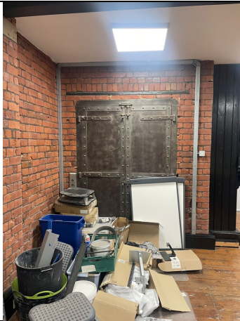
Figure 14: Example of original hoist door.
