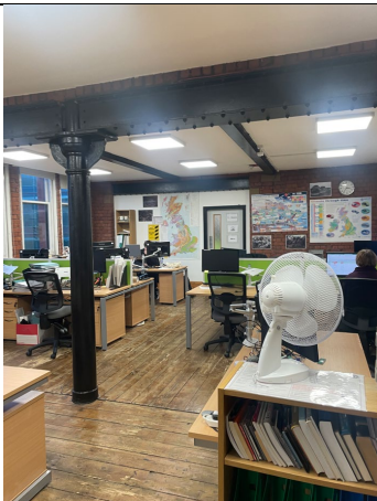
Figure 16: Original exposed flooring, redbrick walls, columns and beams are of high significance. Later alterations and additions such as plasterboard ceilings are of no significance.
