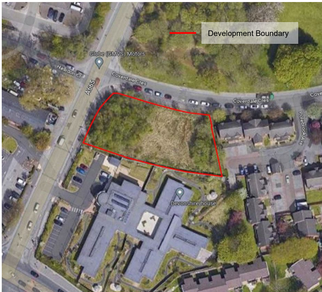
Figure 1: Site Location (Google Maps)
