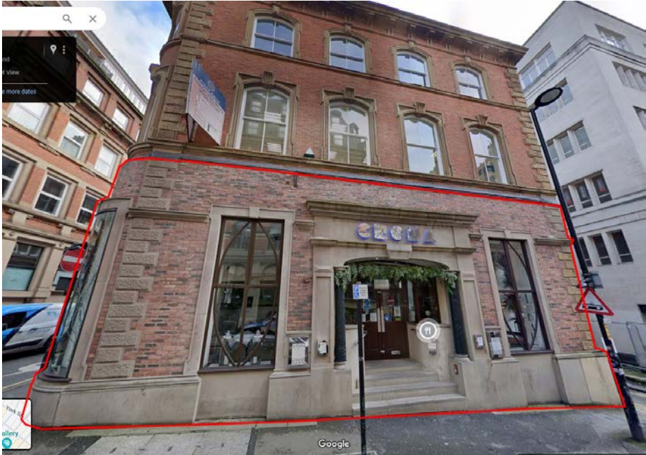
Fig. 02: 1-3 Clarence Street, showing late 90s remodelling at ground floor in non original brickwork
