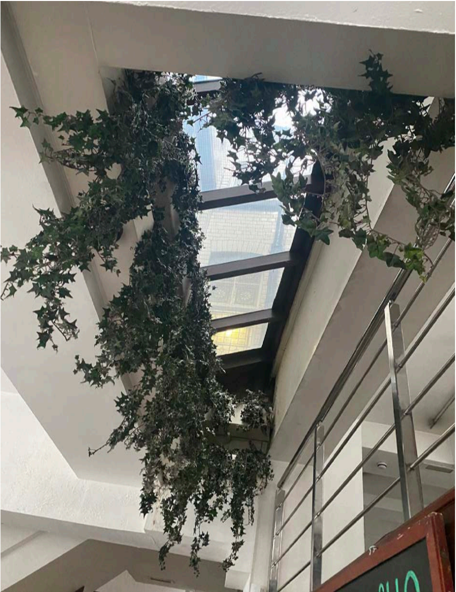
Fig. 16: Internal view of existing rooflight
