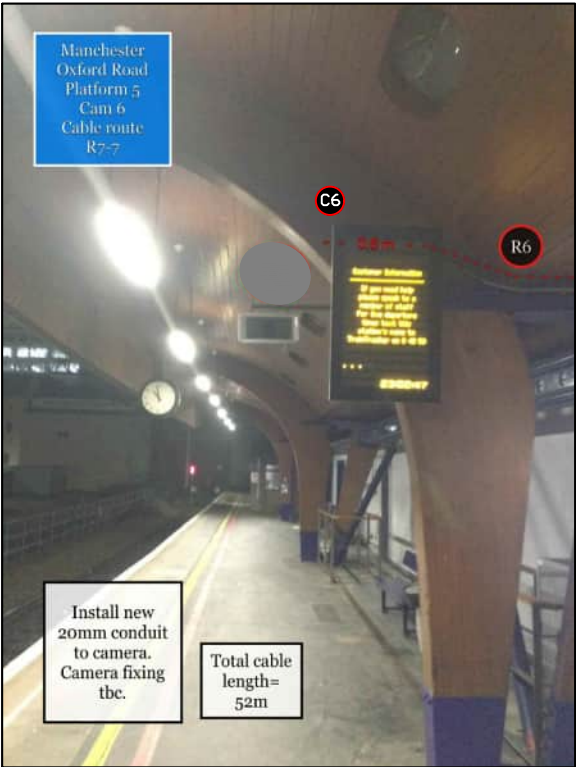
PHOTO 13 NEW 20MM CONDUIT TO BE INSTALLED TO CAMERA 6.
