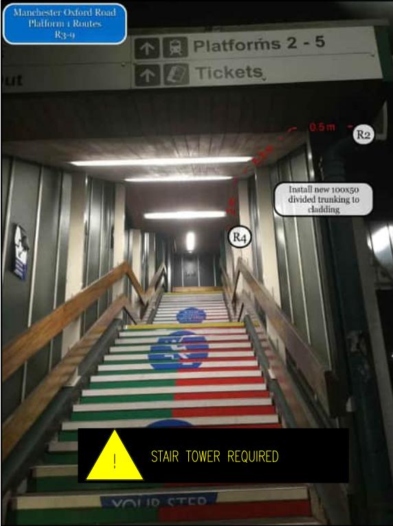
PHOTO 74 NEW 100X50MM TRUNKING TO BE INSTALLED TO CEILING CLADDING ABOVE STAIRS DOWN TO PLATFORM LEVEL.
