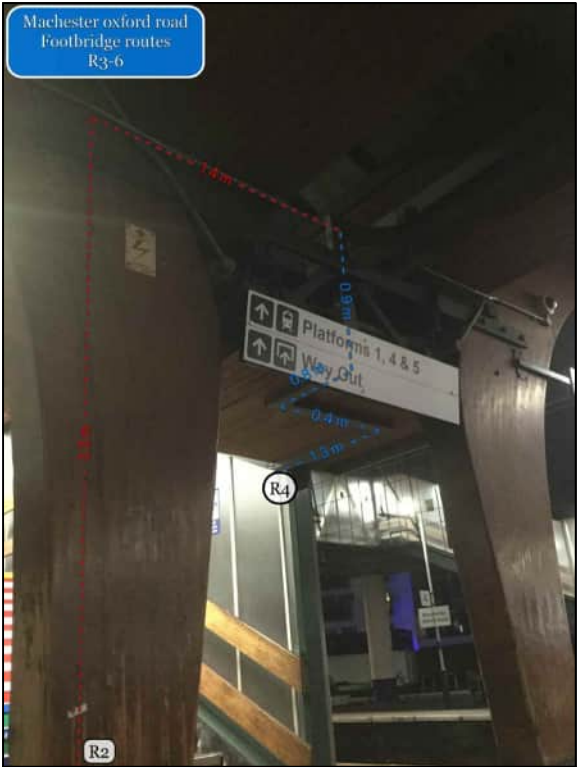
PHOTO 67 INSTALL 150X100MM TRUNKING UP COLUMN AND ACROSS TO LINK WITH EXISTING TRUNKING.
