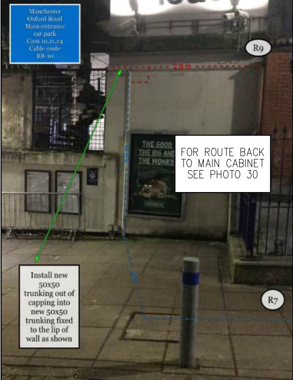
PHOTO 46 NEW 50X50MM TRUNKING TO BE INSTALLED FROM EXISTING CMS.
