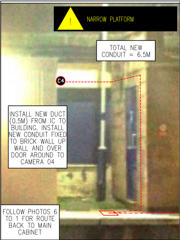
PHOTO 10 NEW 20MM CONDUIT DOWN THE WALL, INSTALL NEW SUB-DUCT TO NEW INSPECTION CHAMBER.
