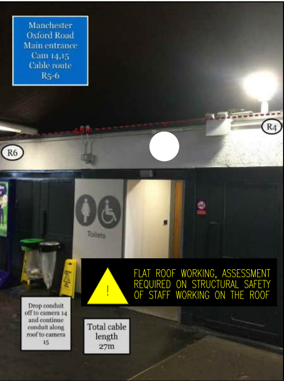
PHOTO 53 CONTINUE NEW 25MM CONDUIT ALONG ROOF TOWARDS CAMERA 15.
