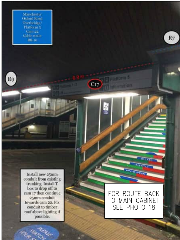
PHOTO 23 NEW 25MM CONDUIT TO BE INSTALLED FIXED TO TIMBER ROOF, FROM EXISTING CMS. CONDUIT T BOX TO BE INSTALLED TO CAMERA 17.
