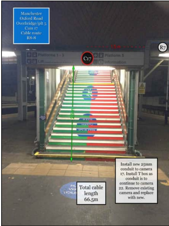
PHOTO 18 INSTALL NEW 25MM CONDUIT FIXED TO WOODEN CEILING TO CAMERA 17.
