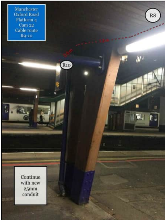
PHOTO 24 CONTINUE 25MM CONDUIT INSTALLATION FORM PHOTO 25.
