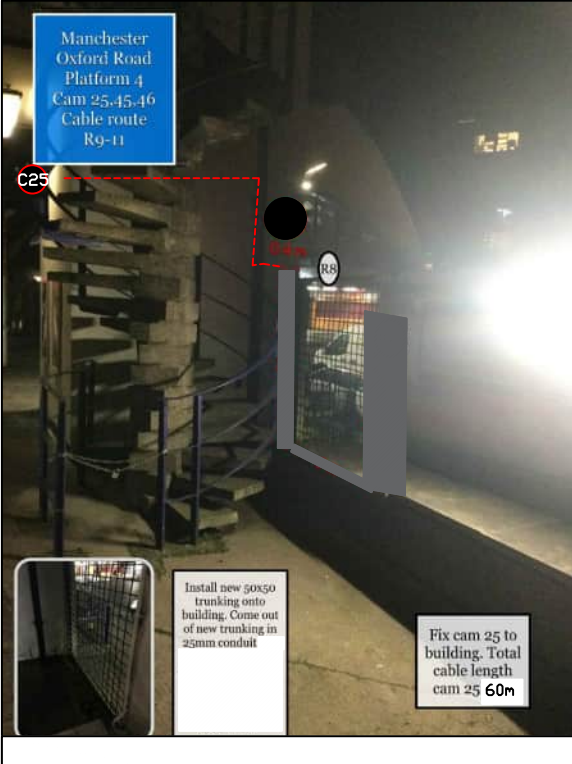
PHOTO 32 NEW 50X50MM TRUNKING FROM PHOTO 31. NEW 20MM CONDUIT TO BE INSTALLED WALL MOUNTED TO CAMERA 25.
