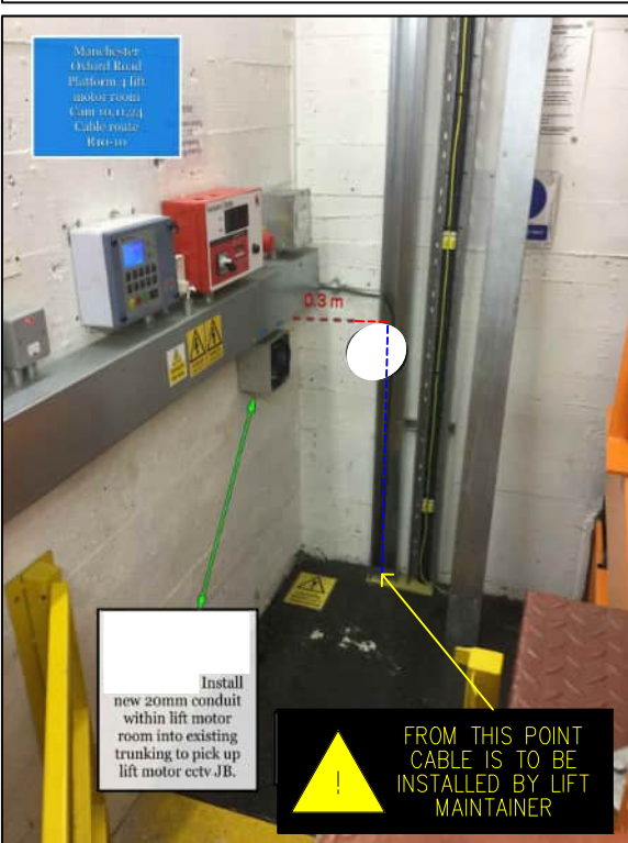
PHOTO 64 NEW CABLE TO BE ROUTED UP THE LIFT SHAFT. FROM EXISTING TRUNKING INSTALL A NEW 20MM CONDUIT TO ADJACENT TRUNKING
