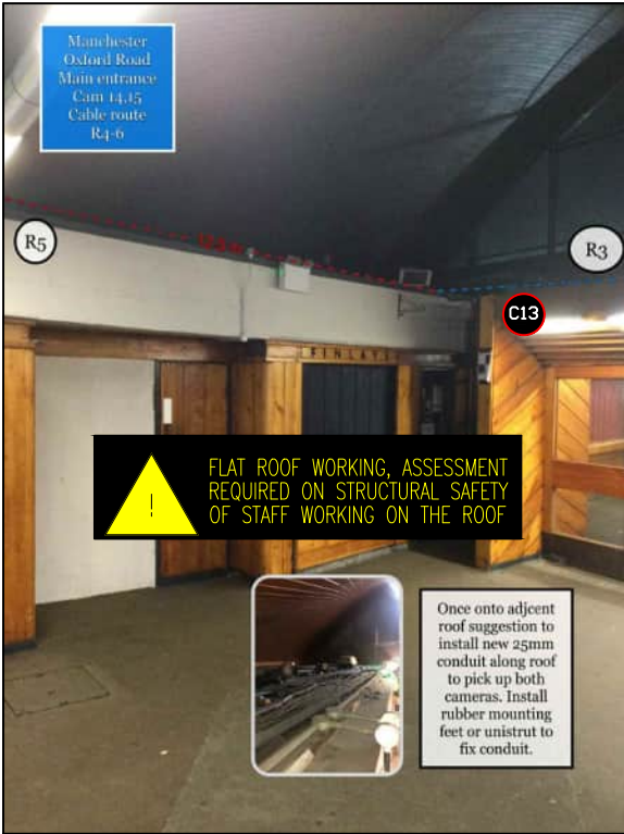
PHOTO 51 NEW 25MM CONDUIT TO BE INSTALLED ON THE ROOF USING MOUNTING FEET, FROM EXISTING CMS.
