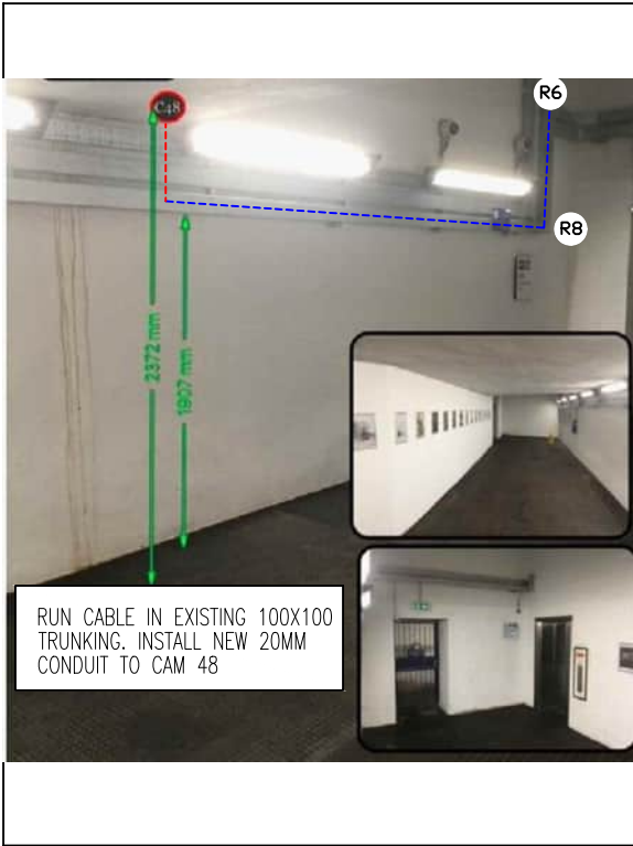
PHOTO 59 INSTALL 20MM CONDUIT FROM EXISTING TRUNKING TO CAMERA 48.
