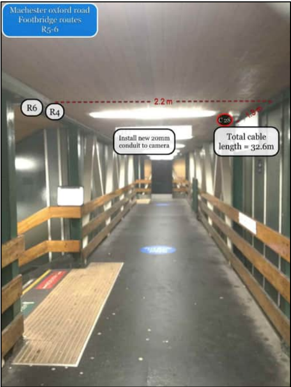
PHOTO 69 INSTALL 25MM CONDUIT FROM EXISTING TRUNKING TO CAMERA 28.
