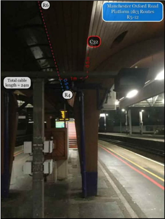
PHOTO 83 NEW 20MM CONDUIT TO BE INSTALLED OFF THE EXISTING CMS TO CAMERA 32.
