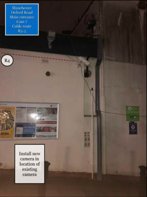
PHOTO 37 NEW 20MM CONDUIT TO BE INSTALLED TO CAMERA 7.
