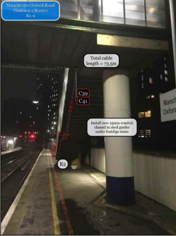
PHOTO 78 INSTALL NEW 25MM CONDUIT TO THE UNDERSIDE OF THE STAIRS, FIXED WITH GIRDER CLAMPS TO CAMERAS 39 & 41.
