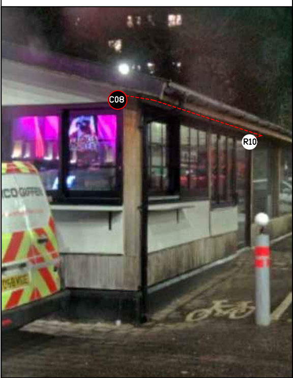
PHOTO 45 NEW 20MM CONDUIT TO BE INSTALLED OUT OF THE CYCLE CENTER AND ROUTED THE OUTSIDE OF THE CAFE TO CAMERA 8.
