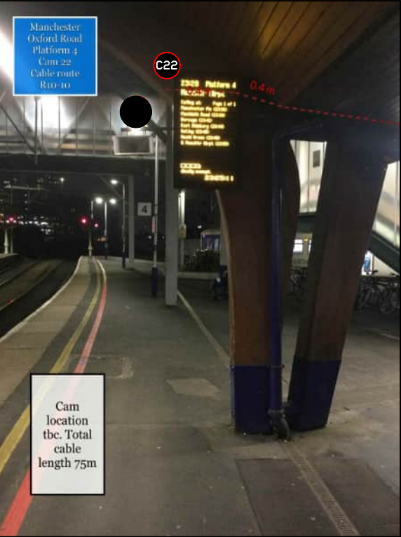
PHOTO 25 CONTINUE 25MM CONDUIT FROM PHOTO 26 TERMINATING AT CAMERA 22.
