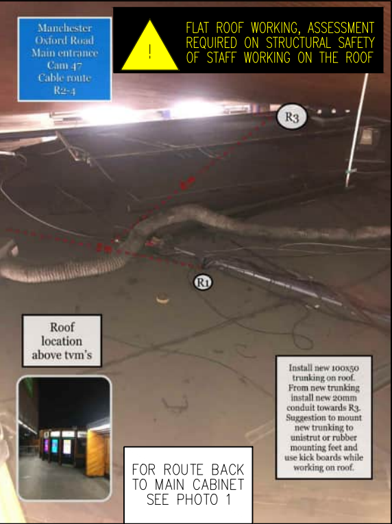
PHOTO 33 NEW 20MM CONDUIT TO BE INSTALLED FROM NEW 100X50MM TRUNKING.
