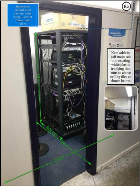
PHOTO 1 NEW FLEXIBLE KOEPEX TO BE USED TO TRANSITION BETWEEN EXISTING CABINET TOP AND EXISTING PLASTIC TRUNKING.
