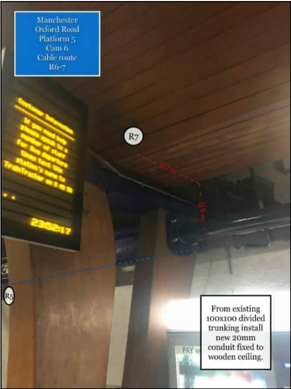
PHOTO 12 NEW 20MM CONDUIT TO BE INSTALLED FROM EXISTING TRUNKING FIXED TO WOODEN CEILING.
