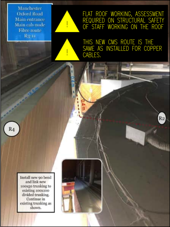
PHOTO 3 NEW 100X50MM TRUNKING TO BE INSTALLED TO MEET EXISTING.
