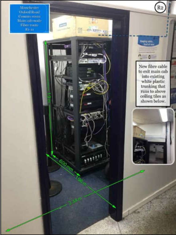
PHOTO 1 NEW FLEXIBLE KOPEX TO BE USED TO TRANSITION BETWEEN EXISTING CABINET TOP AND EXISTING PLASTIC TRUNKING.
