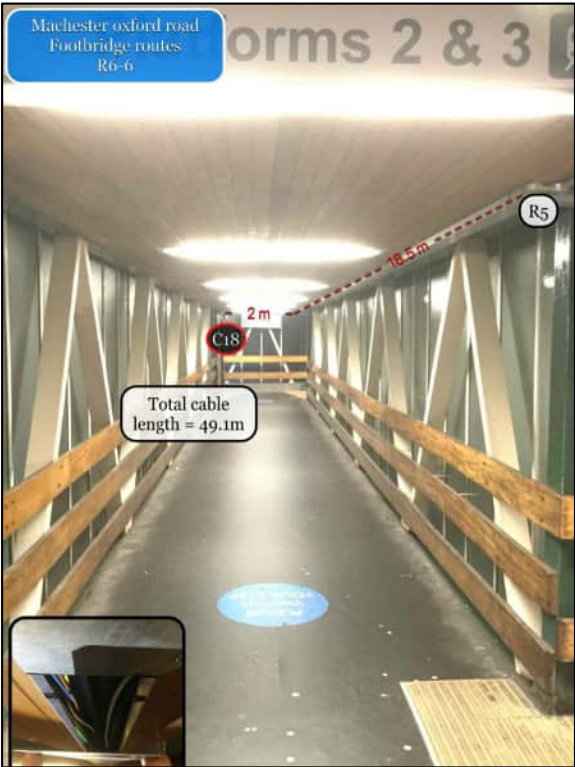
PHOTO 70 INSTALL 20MM CONDUIT FROM EXISTING TRUNKING TO CAMERA 18.
