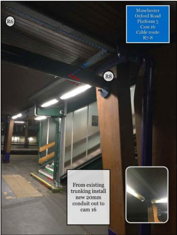
PHOTO 15 NEW 20MM CONDUIT TO BE INSTALLED FROM EXISTING TRUNKING TO CAMERA 16.
