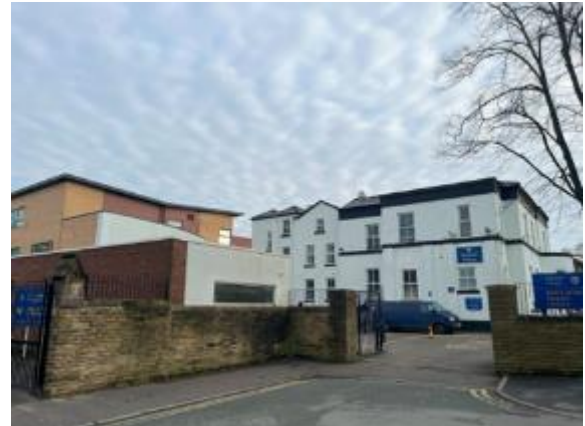
Figure 2.3 The Ryken Building to the left with Sunbury Hall to the right
