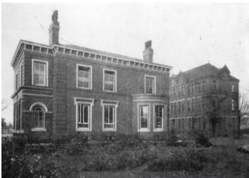
Figure 3.4 Sunbury House before the current render scheme. Note the lost chimney stacks and bracketed eaves. The rear of the Xaverian Building is in the distance.
