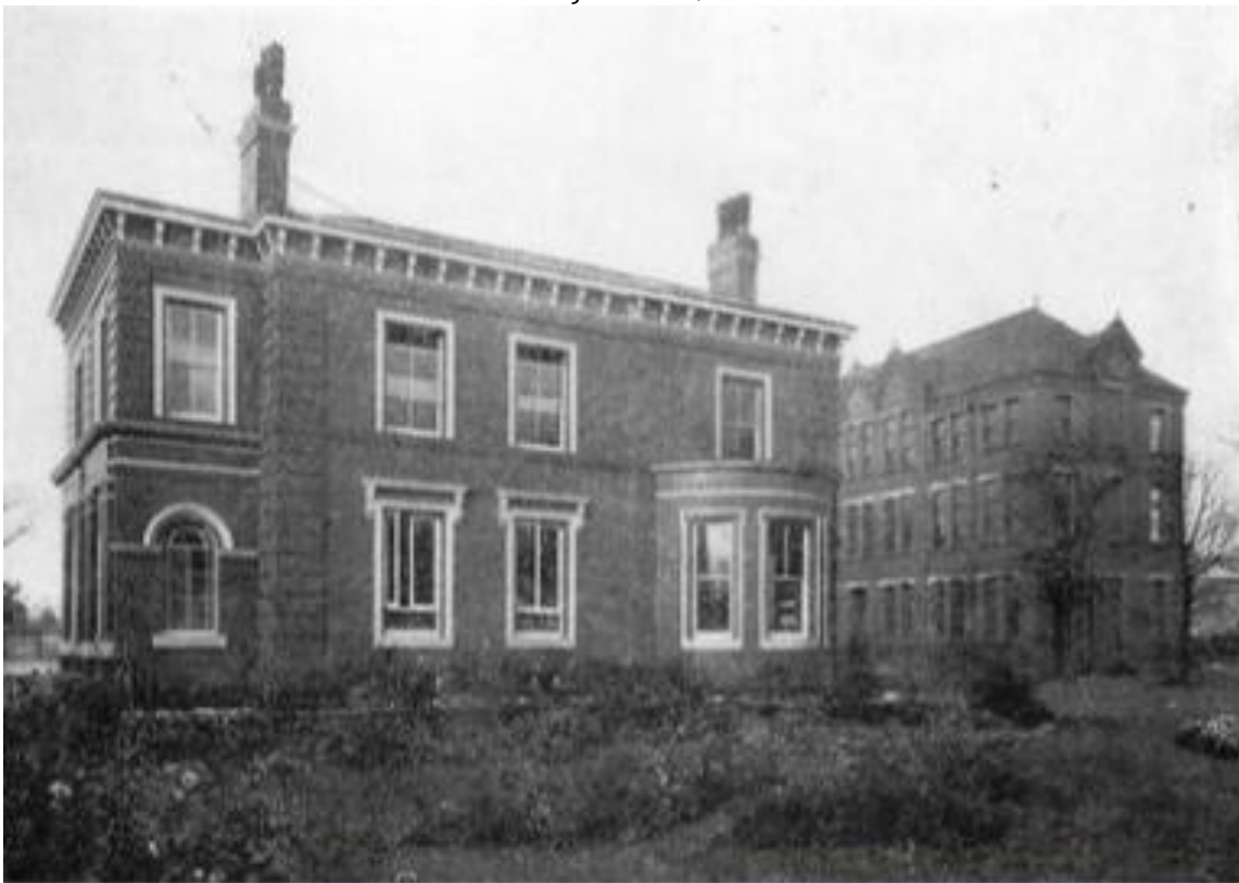
Sunbury House before the current render scheme. Note the lost chimney stacks and bracketed eaves. The rear of the Xaverian Building is in the distance.
